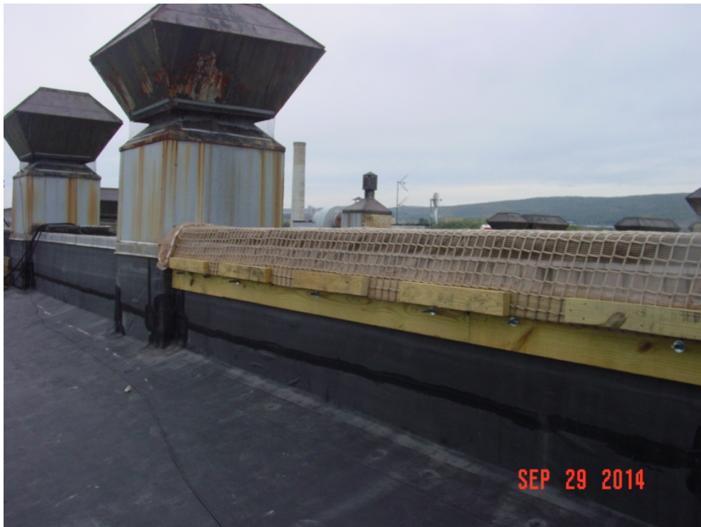
Anchorage of containment netting on rear of existing parapet.
