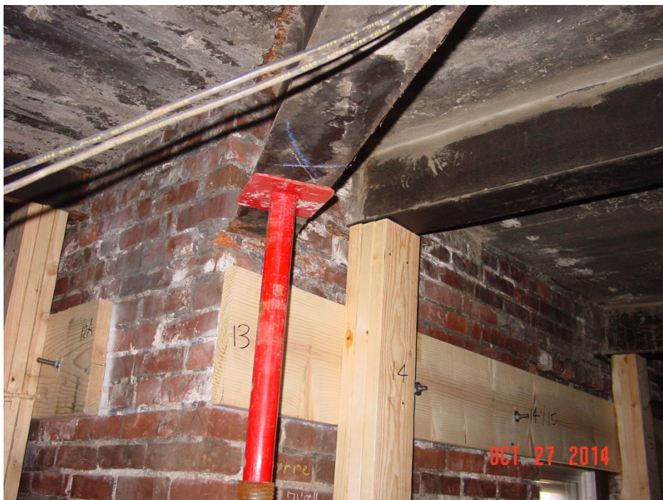
Roof shoring installed in Attic during 2014 courtyard wall repair and containment project
