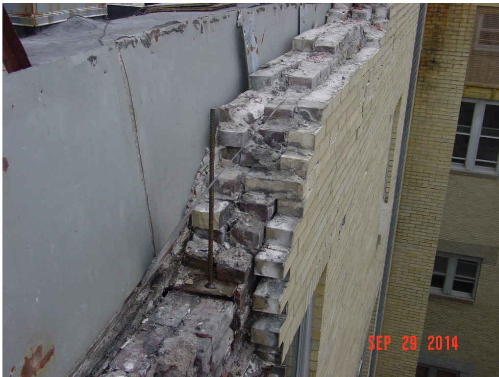
Parapet Steel Reinforcing Bars Added During Courtyard Wall Repairs.
