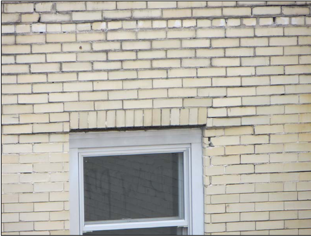
Photograph 39: Corrosion of the window lintels is causing the brick cracking and displacement.
