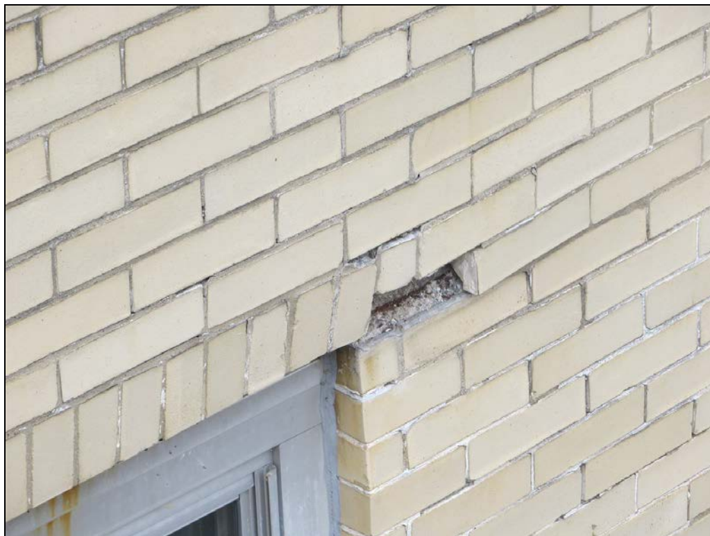
Photograph 41: At this lintel a brick was pushed off the wall from the corroding lintel.
