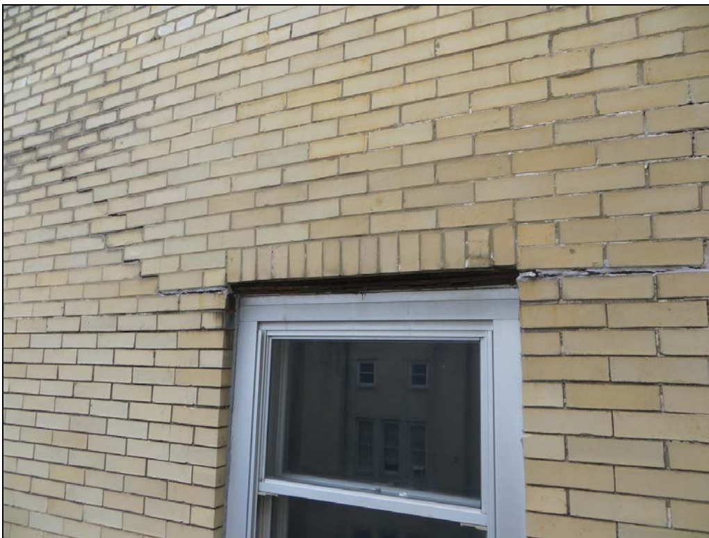
Photograph 40: The heavy corrosion of the lintels caused substantial damage to the surrounding masonry.
