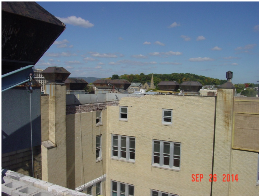
Badly damaged sections of the Courtyard parapets were removed and rebuilt in the 2014 repair/containment project.
