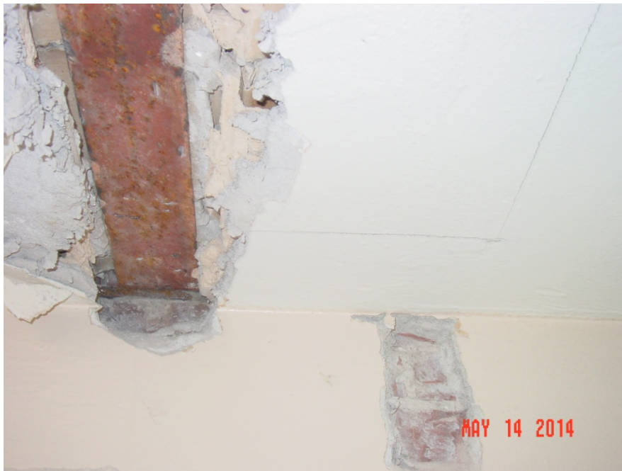
Interior 4th floor beam bearing on Courtyard wall was exposed and found to be in sound condition.
