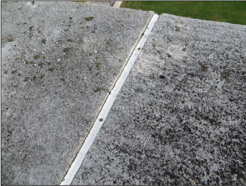
Photograph 15: Most of the sealant joints between the coping pieces were failed.
