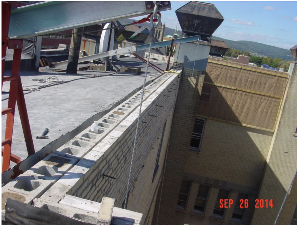
View of re-built section of parapet during 2014 repair/containment project.
