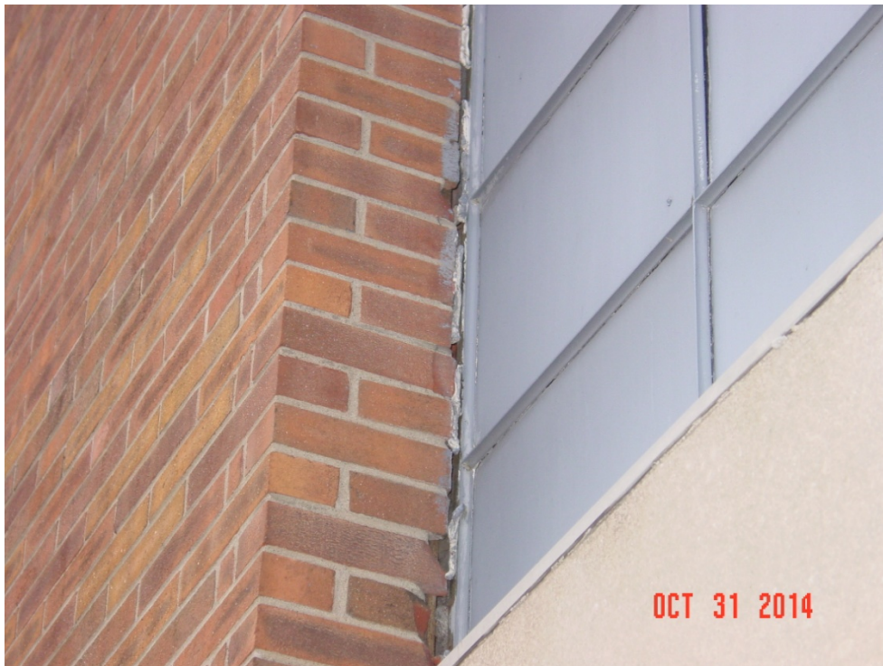
Brick / window joint on south wall of Gymnasium. Joint is failing and allow water to infiltrate which may be initiating internal corrosion. The Annex façade should be maintained if short or long-term continued occupancy is anticipated.
