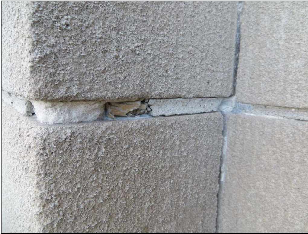
Photograph 11: An original wood shim at a failed mortar joint.
