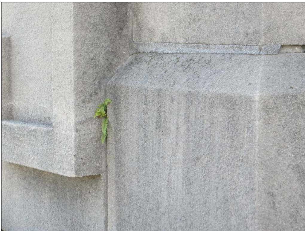
Photograph 12: More plant growth in an open mortar joint.
