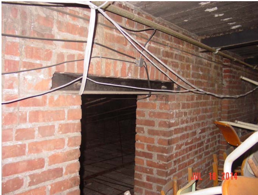
Existing interior Attic brick walls and steel lintels are in sound condition.
