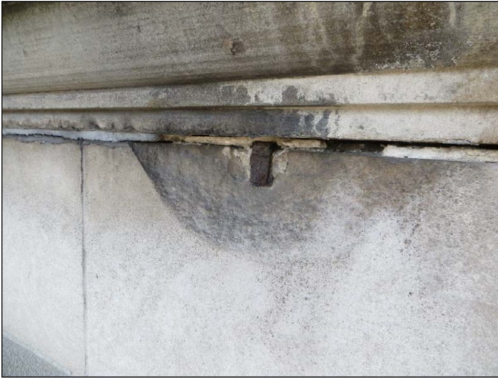
Photograph 19: Most of the anchors at the spall locations were heavily corroded.
