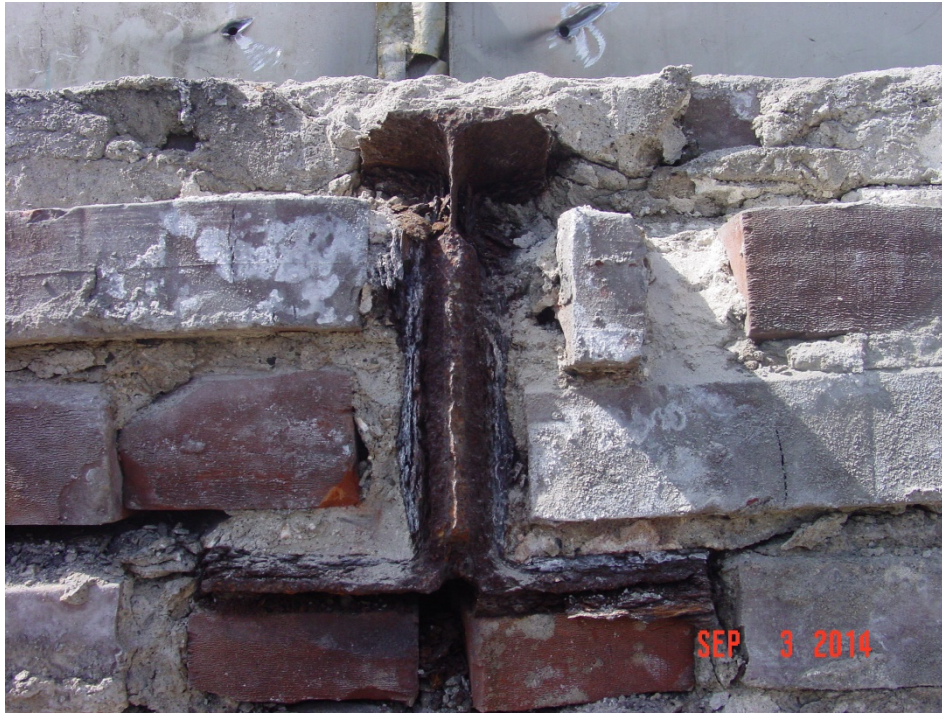
Exposed End of typical roof beam at courtyard wall.
