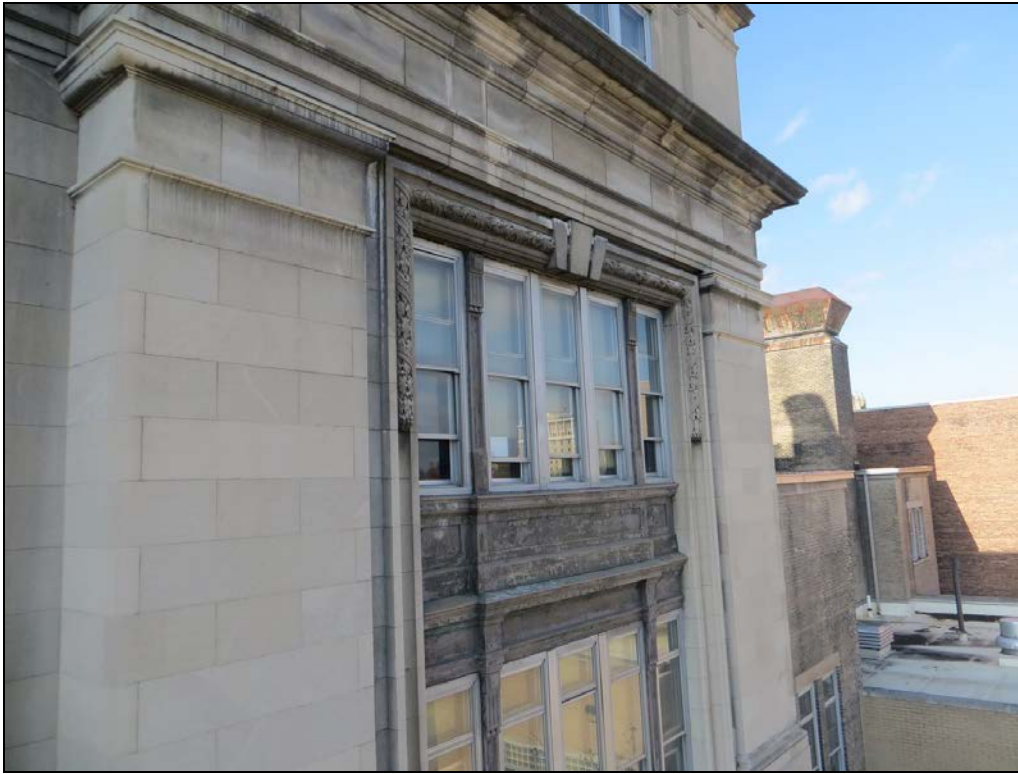
Photograph 43: Copper sheet metal over wood framing was used at the large windows at the end of each elevation.
