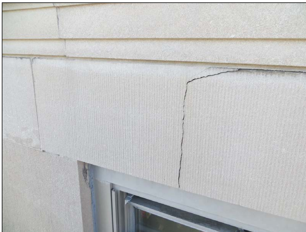
Photograph 24: Some of the cracks were significant, indicating the stone was under significant stresses caused by the corrosion of the steel below.
