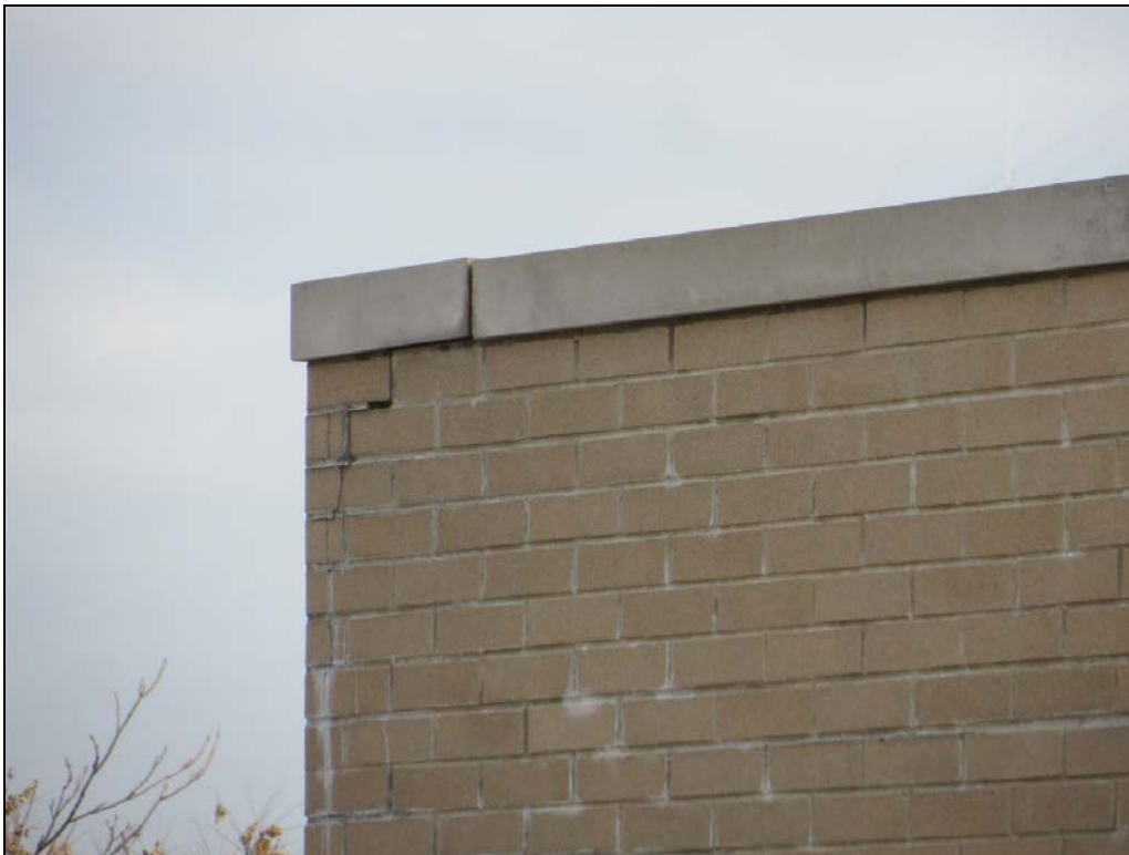
Photograph 34: The chimney was in fair condition, but we did not some cracking and displacement at the upper corner.
