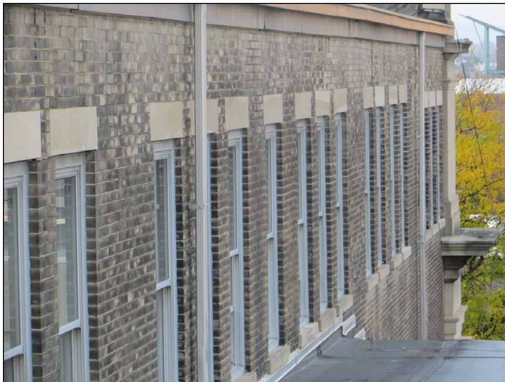
Photograph 31: View of the rear elevation of the building. Note the stone lintels over the window openings.
