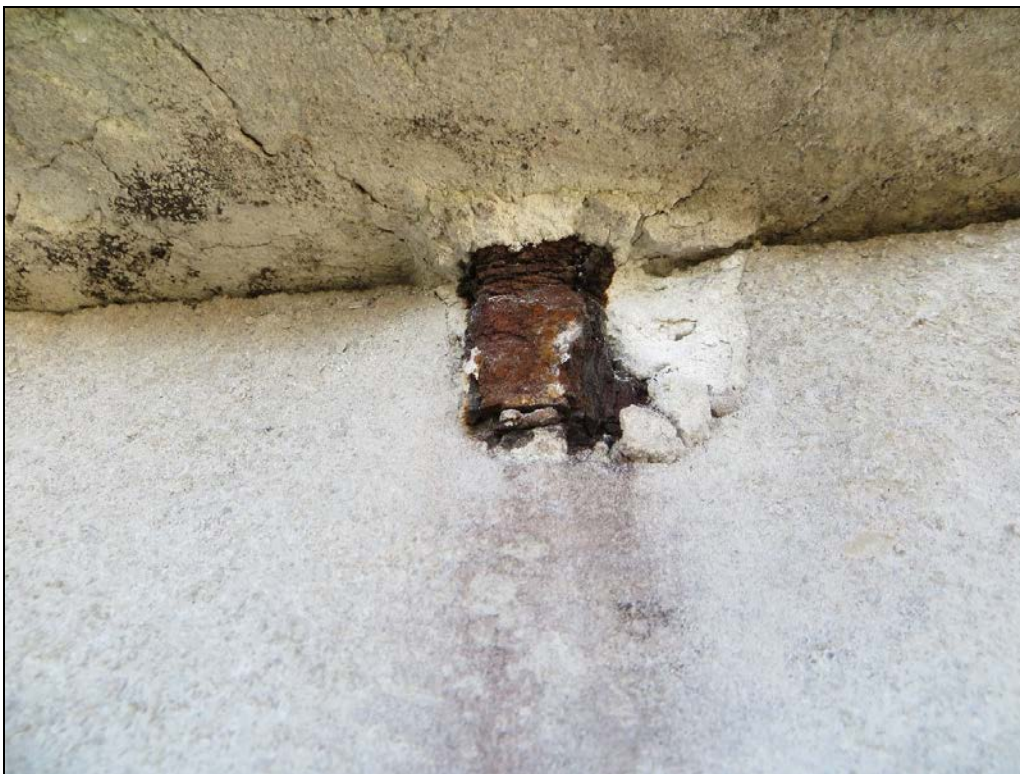
Photograph 20: The corrosion of the anchors is caused by water within the wall. As the walls take on more water the rate of corrosion of the anchors increases.
