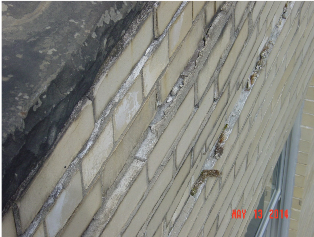
Brick at top of southeast corner of Courtyard wall prior to repairs
