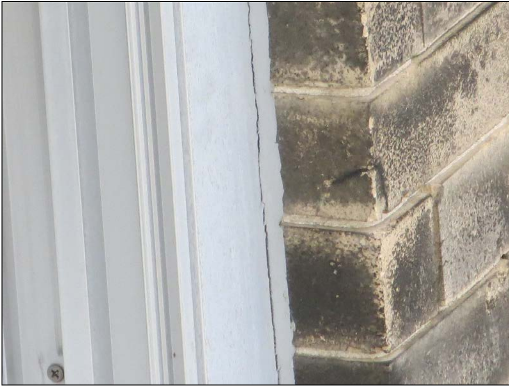
Photograph 49: Failed sealant on the rear elevation of the building.
