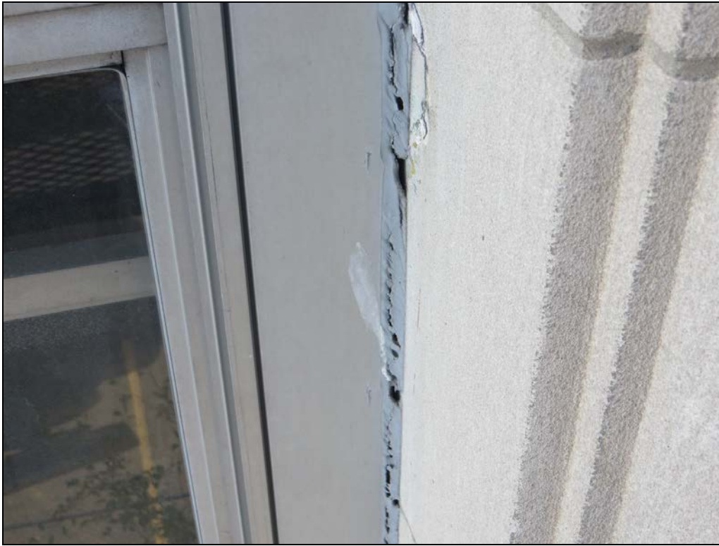
Photograph 45: Failed sealant at the window perimeter.
