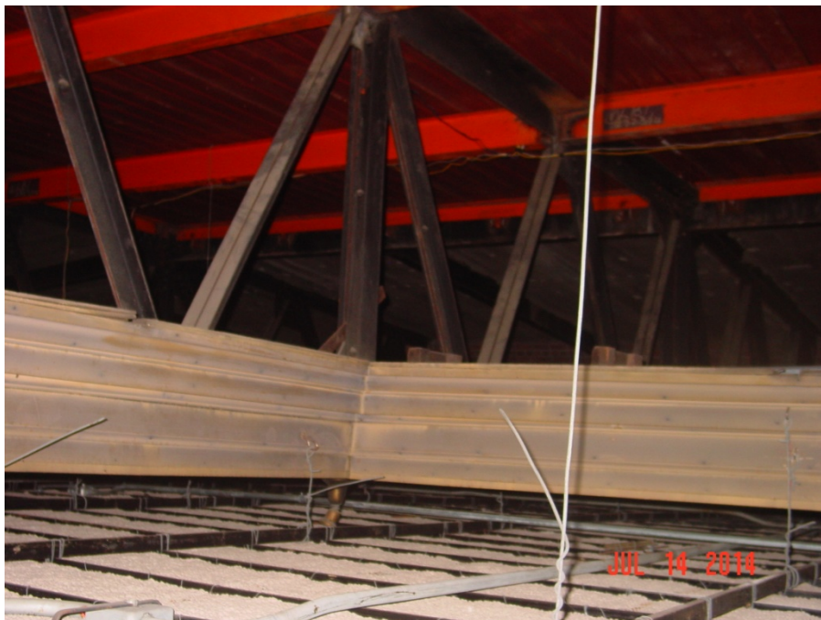
View of former Library skylight window frames and the replacement plaster ceiling hung below.
