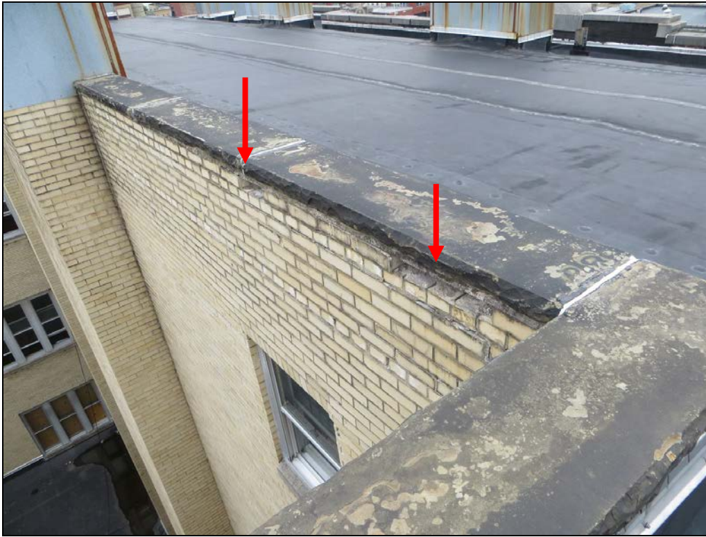
Photograph 37: The brick veneer on the courtyard elevations was in poor condition, particularly at the parapets. Note the missing brick under the coping.
