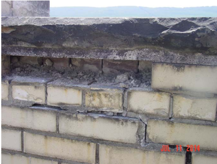
Top of Courtyard parapet prior to repairs in Summer of 2014. Note the deteriorated mortar. The missing bricks were easily removed by hand.
