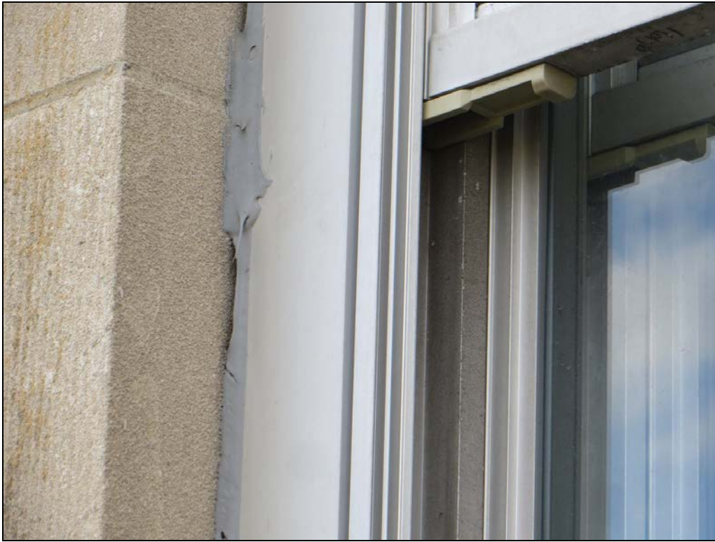
Photograph 47: Poorly installed sealant has lost adhesion to the stone.
