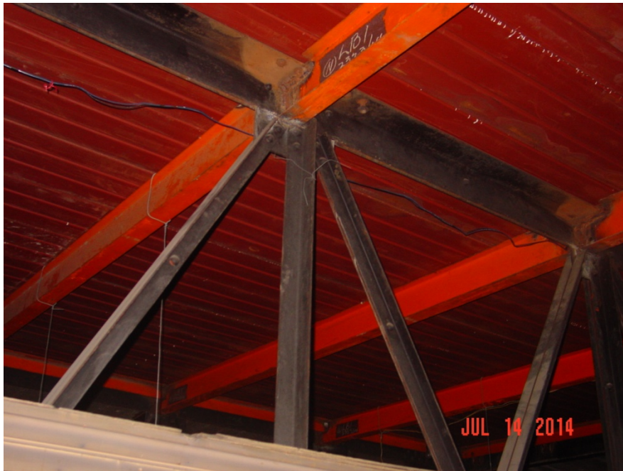
View above library ceiling showing steel framing (orange) in-filled above original skylight.
