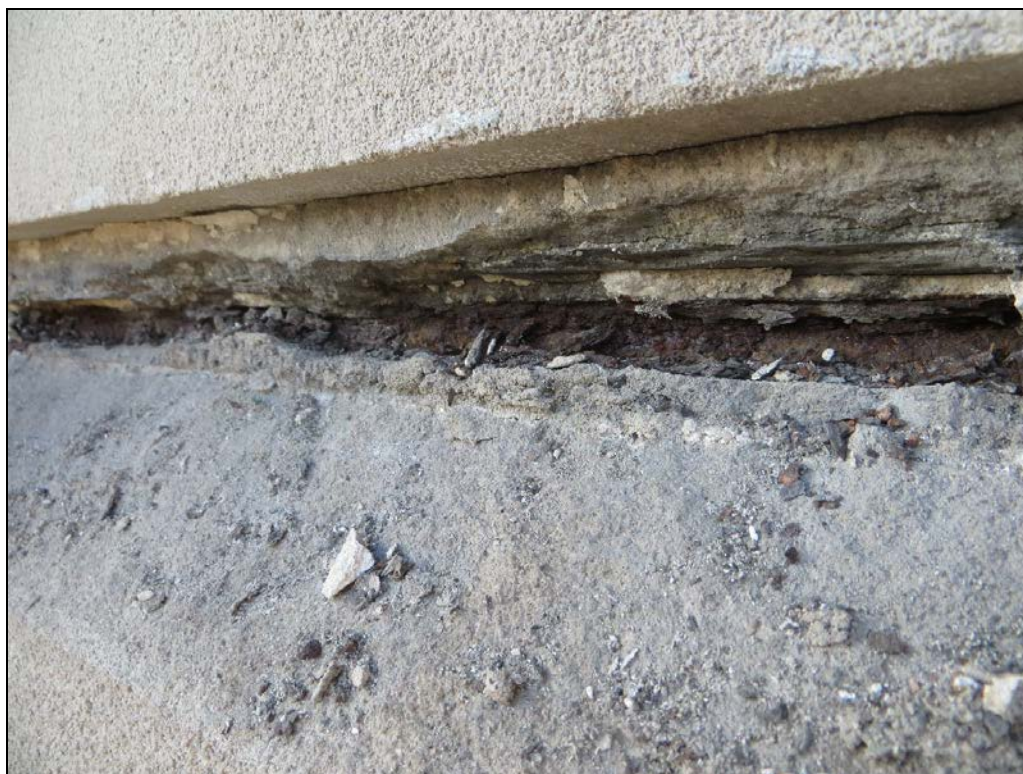
Photograph 30: The steel behind the molding piece was heavily corroded.
