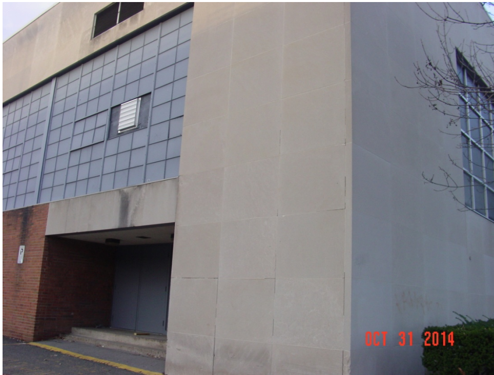
Southeast corner of Annex (Gymnasium). Note the loss of mortar is numerous stone panel joints.
