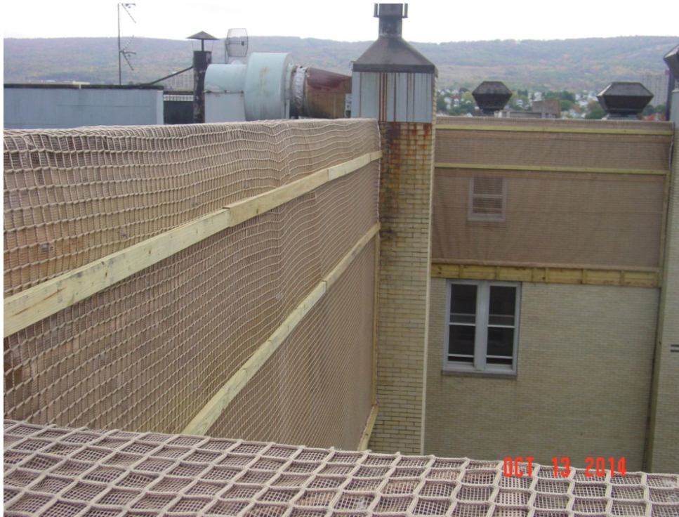
View of completed containment netting installation.
