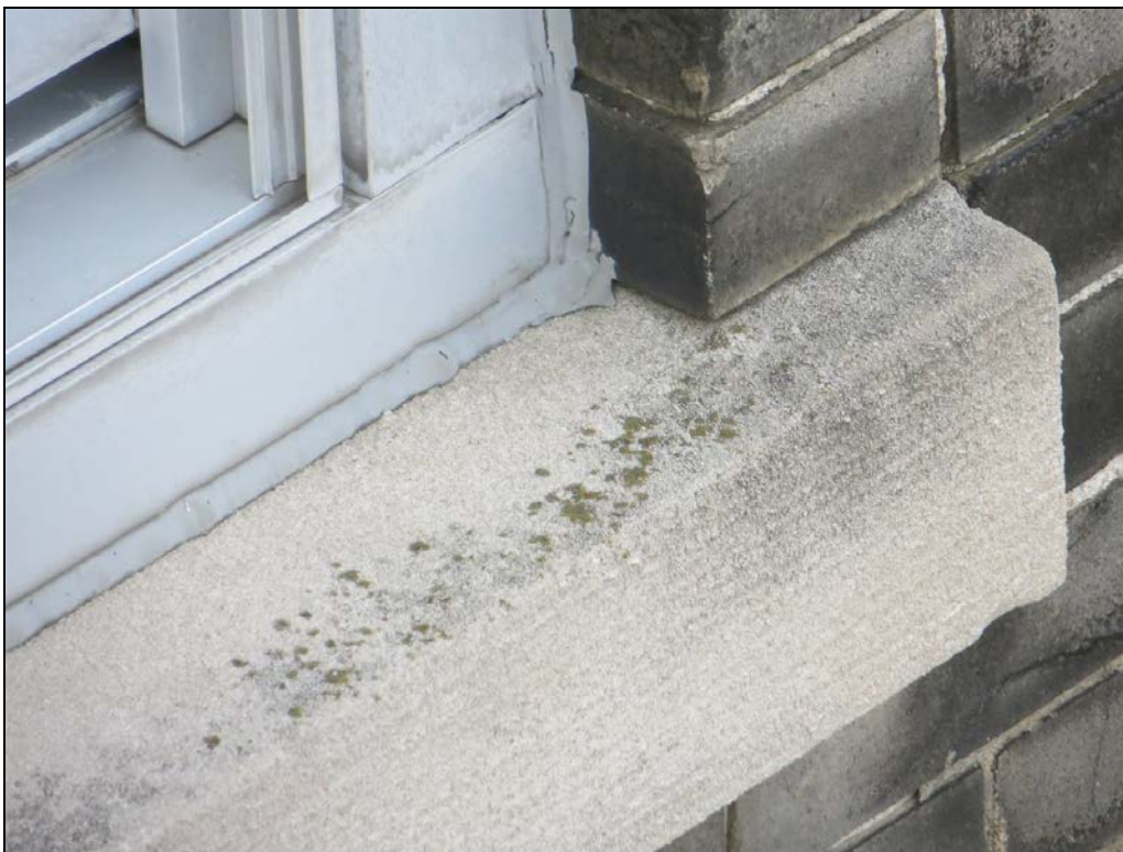
Photograph 50: Sealant on the window sill was never properly tooled, greatly reducing the performance of the sealant.
