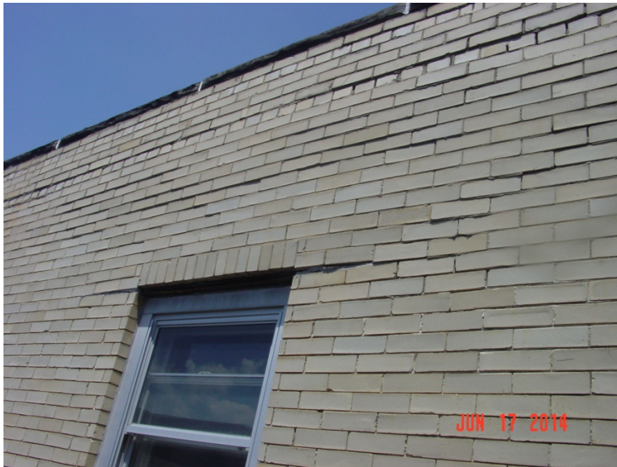
Bowing of brick above an Attic window due to corrosion and expansion of the steel lintel.
