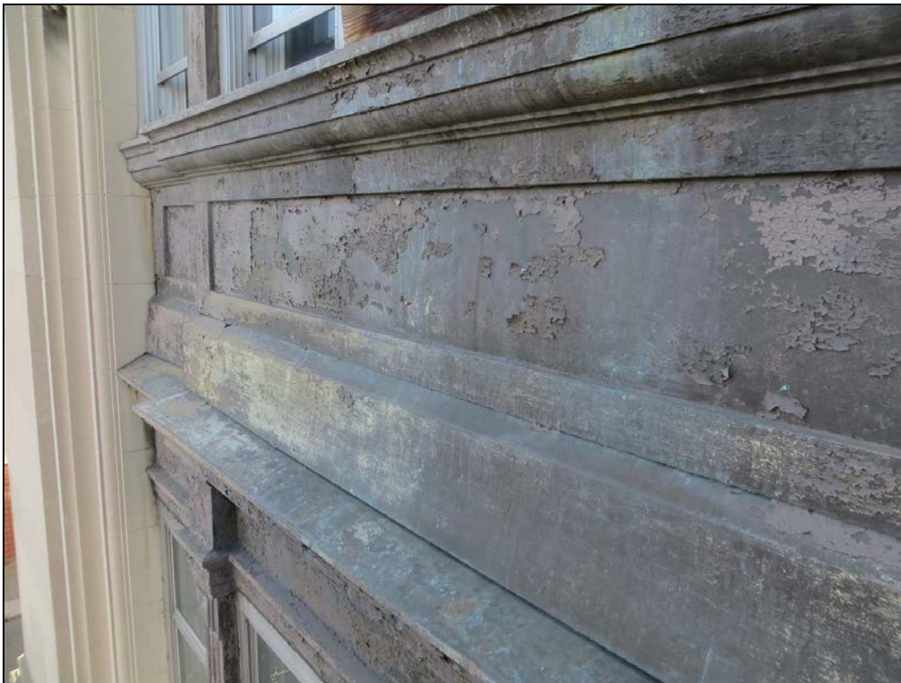
Photograph 44: The copper sheet metal was painted. The paint is now peeling at most locations.
