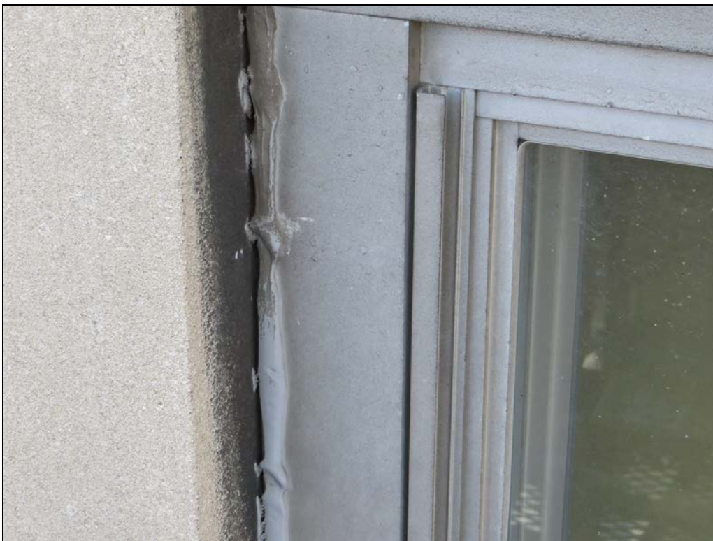
Photograph 48: Sealant has failed the entire height of the window jamb.
