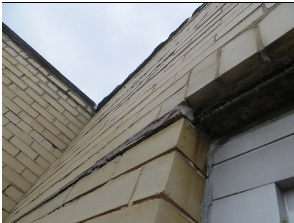
Photograph 42: The brick above the lintel has displaced outward.
