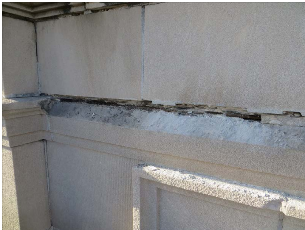
Photograph 29: The entire molding piece was removed by hand without the use of any tools.
