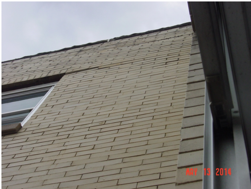
Courtyard wall prior to 2014 repairs. Note top corner of window where heavy corrosion in steel window lintels caused the steel to delaminate, expand and push the brick outwards.
