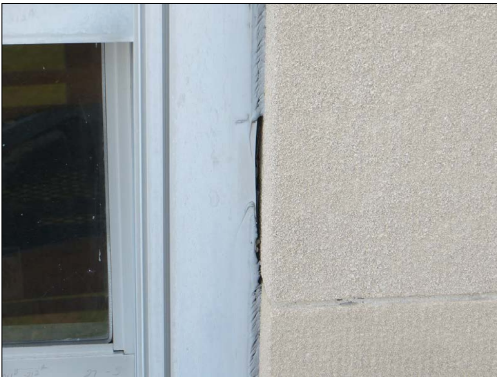
Photograph 46: Sealant was not installed at a section of the window perimeter.
