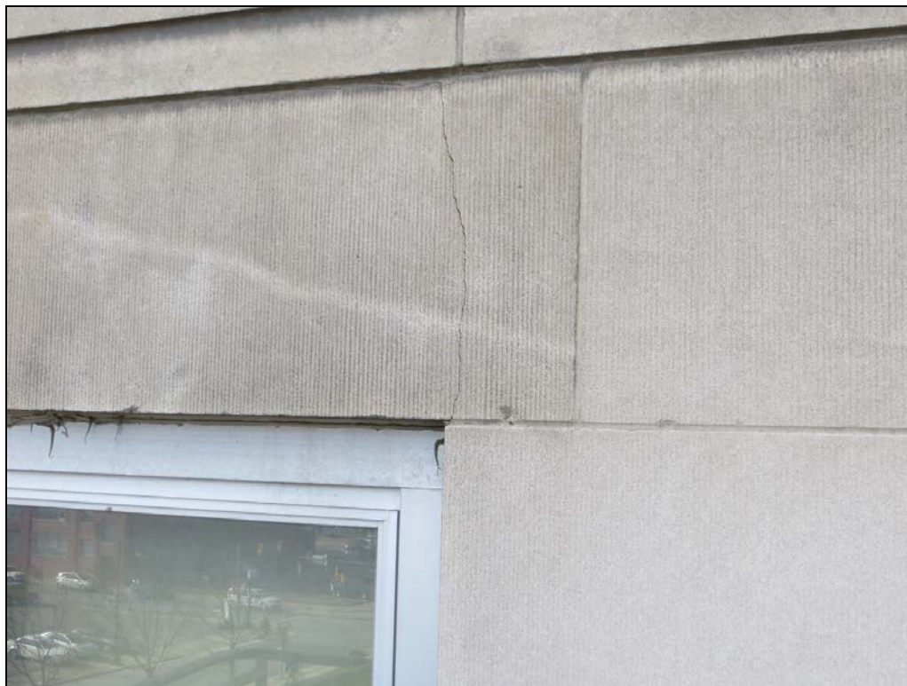
Photograph 23: Cracked stone pieces were noted above some of the windows.
