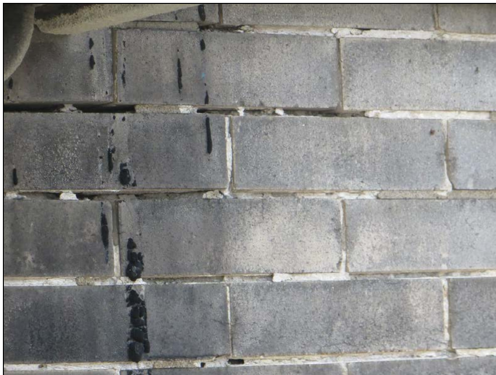
Photograph 35: The mortar joints on the rear of the building were in poor condition.
