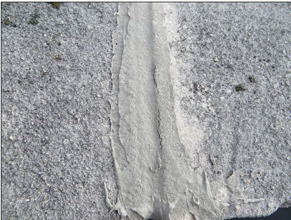
Photograph 16: Even newly replaced sealant joints were already beginning to fail.
