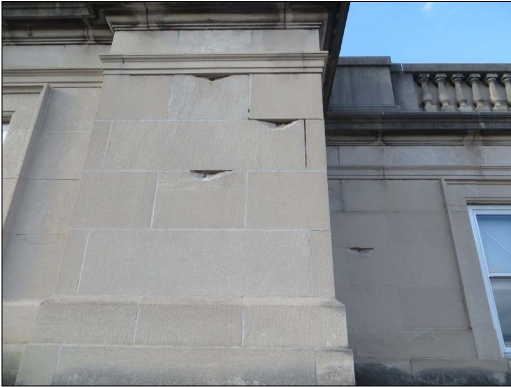
Photograph 5: Multiple spalls in close proximity to each other.
