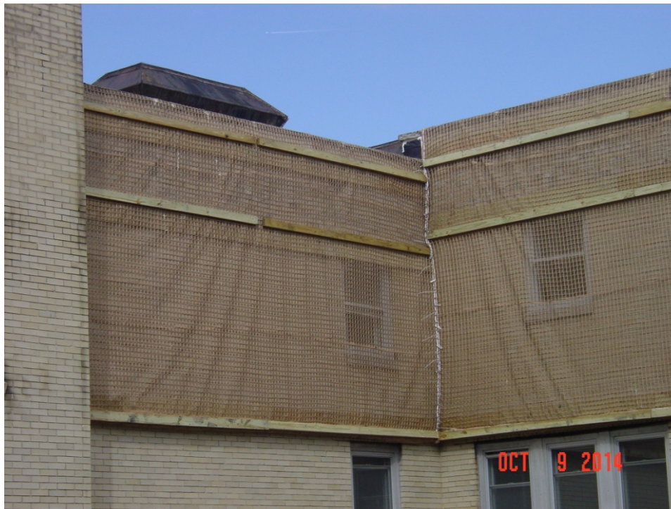
View of completed repair/containment netting in northwest corner of Courtyard. Existing parapet was rebuilt at lower elevation on west side where roof elevation drops above Auditorium stage.
