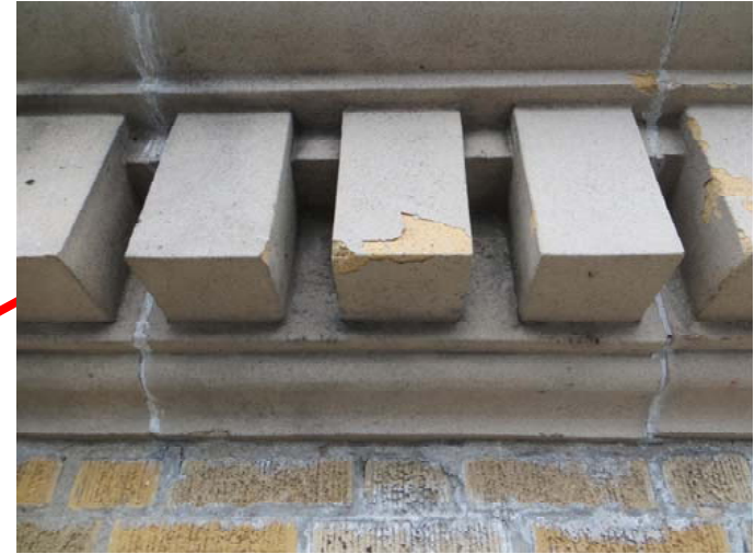
Spalling of the glazing was present at a few locations in this area.
