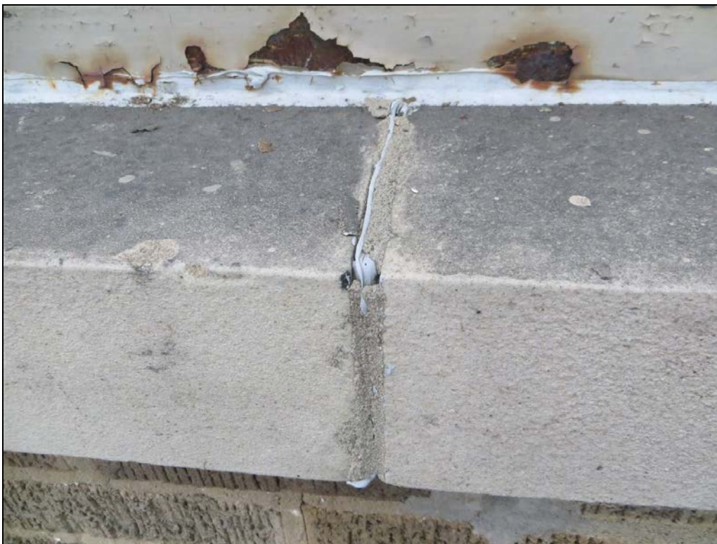
Photograph 42: The failures of the window sill joints are allowing excessive amounts of water in the wall assembly.
