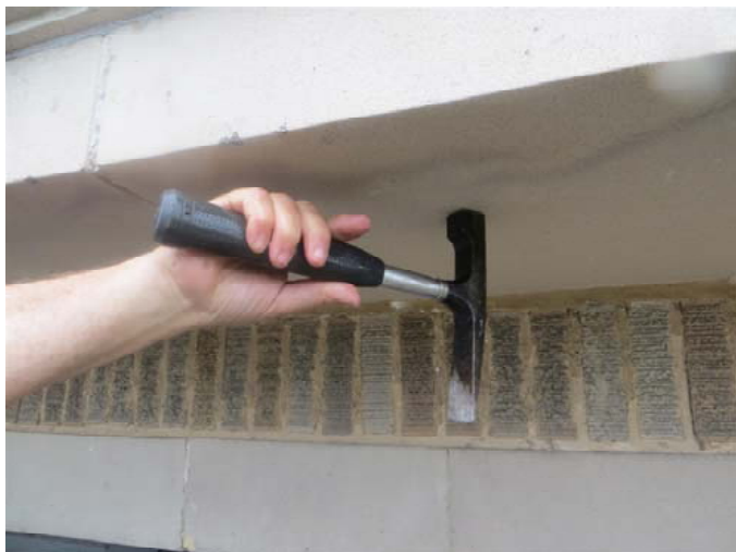
All of the terra cotta pieces were sounded. We did not find any pieces that were unstable or significantly displaced
