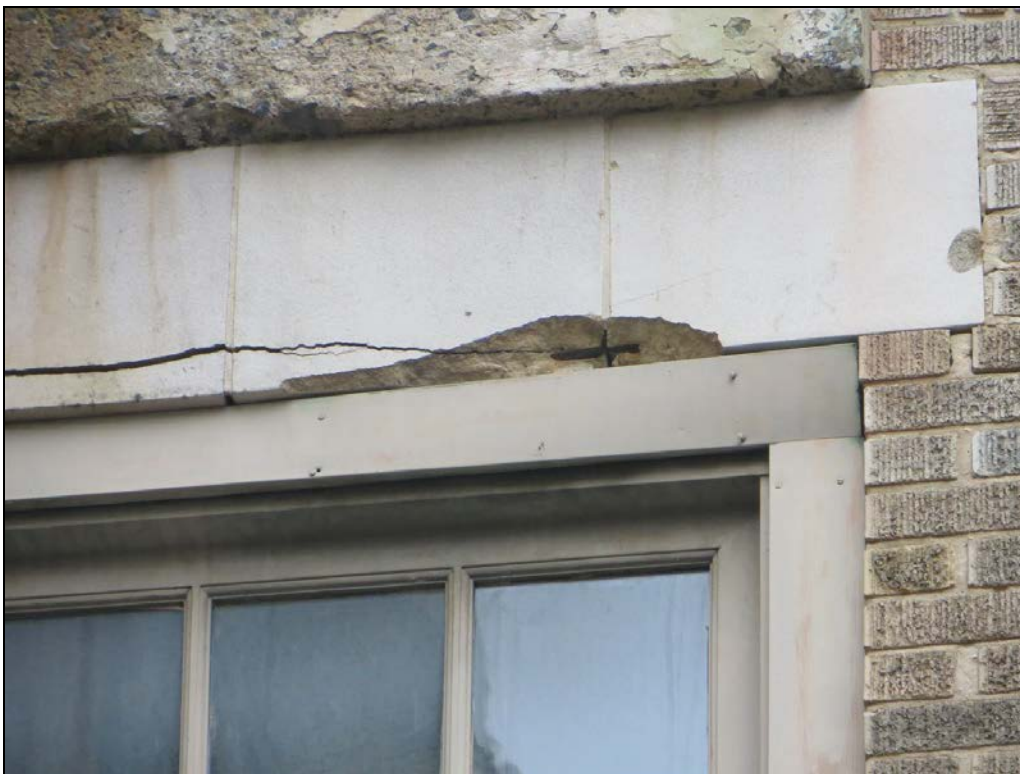
Photograph 38: Large spall and crack in the window header pieces. Additional terra cotta pieces will eventually fall to the ground.
