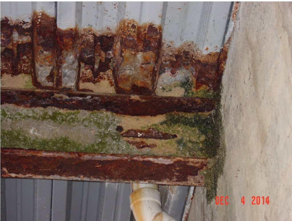
Corroded steel beam under the north end walkway. Fireproofing on this beam has failed and fallen from beam. Remnants of the fireproofing remain on the beam web with moss growth, indication high moisture content.
