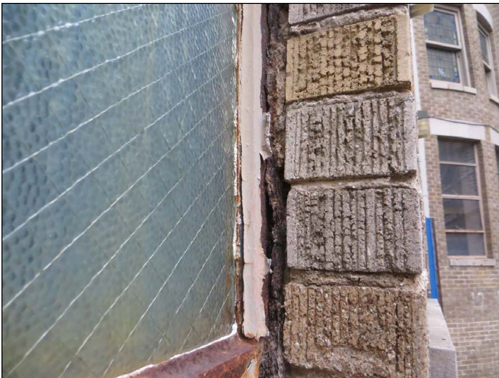
Photograph 58: The steel frames of the original windows are built into the surrounding masonry and may have been used to temporarily support the terra cotta above. Extensive masonry work will be required when the steel frames are removed.
