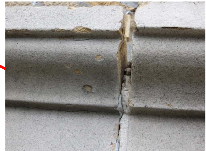
Sealant was installed over the majority of the terra cotta mortar joints. The sealant and mortar had failed at most locations.
