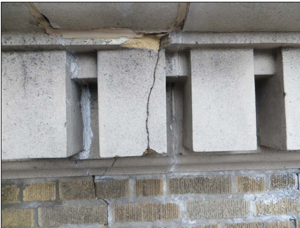
Photograph 26: Cracked dentil piece that will eventually break loose and fall to the ground.
