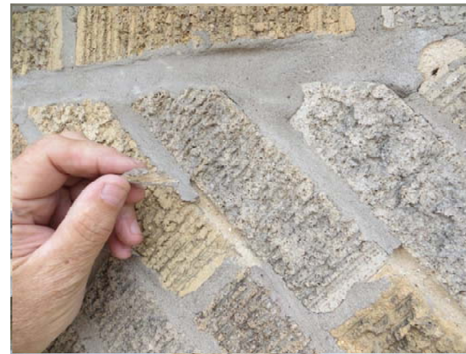
Several attempts to repoint the mortar were improperly completed and have failed.
