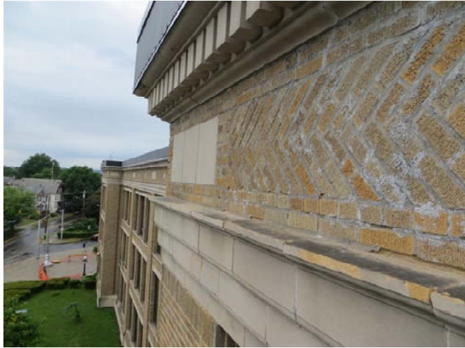
Efflorescence (white staining) was present at several sections of brick, a sign that the masonry is drying out.
