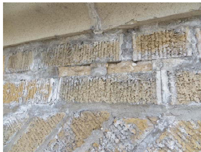
Failed mortar joints directly below the terra cotta dentil.
