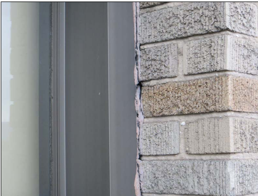
Photograph 50: The failed sealants are allowing large amounts of bulk rain water to enter the exterior wall assembly.
