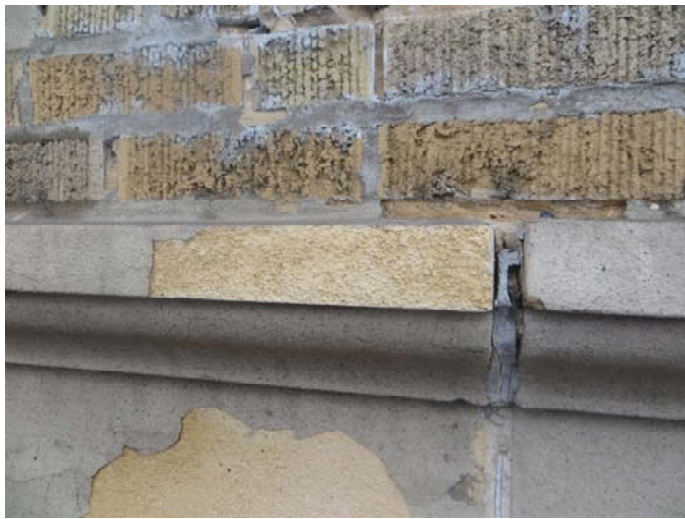
Spalling of the glaze was present at many locations.
