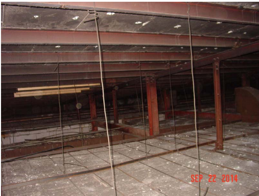
Main Building roof framing visible in attic above Hanover Street side.
