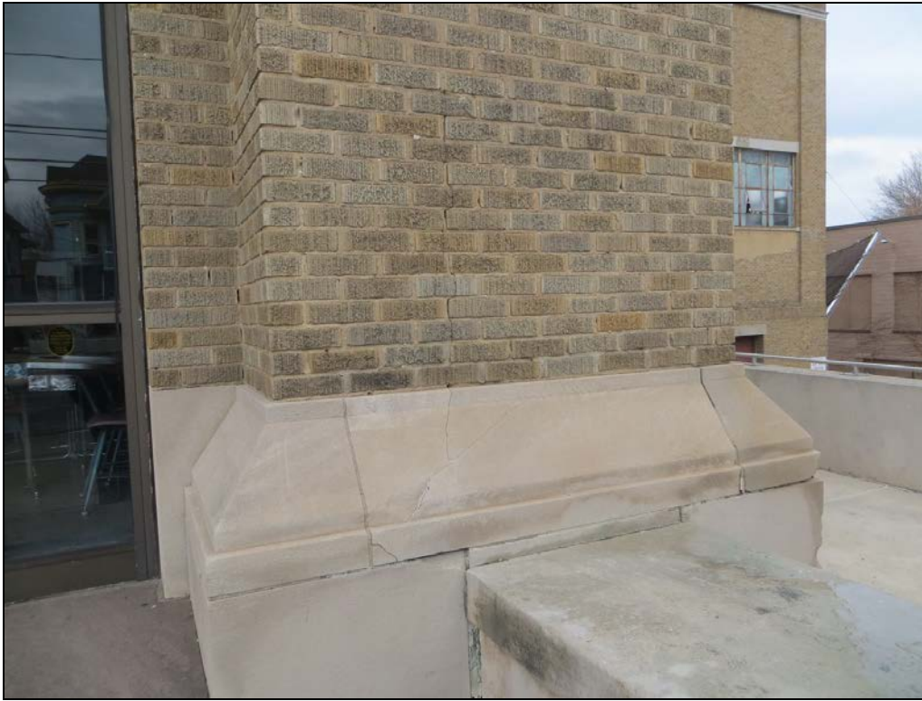
Photograph 45: Cracked limestone piece at the base of the building.
