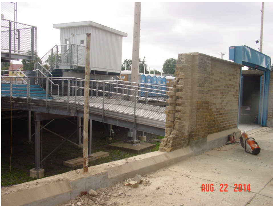
Deteriorated brick wall removal near Old River Road stadium entrance. The section was replaced with chain link fencing.
