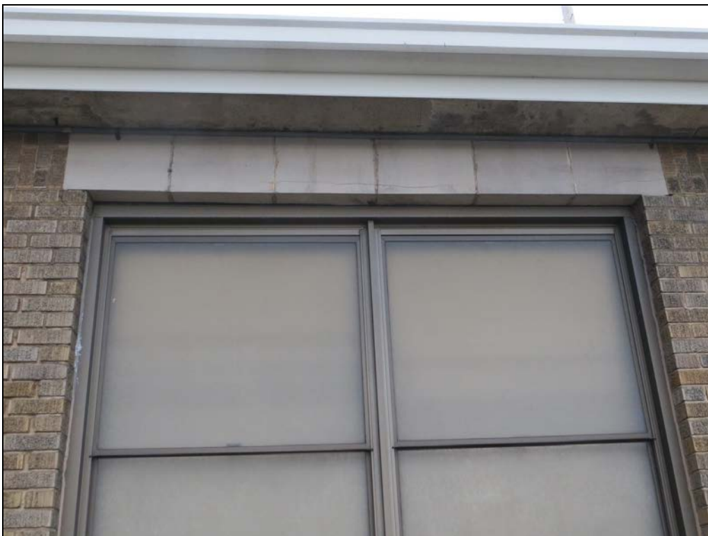
Photograph 56: New retrofit windows were installed over the original steel frames at many locations.
