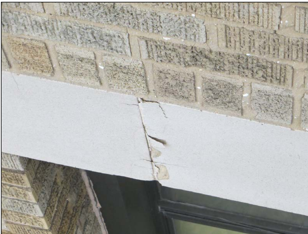
Photograph 40: The spalling is an indication the terra cotta is overstressed, typically caused by thermal expansion.
