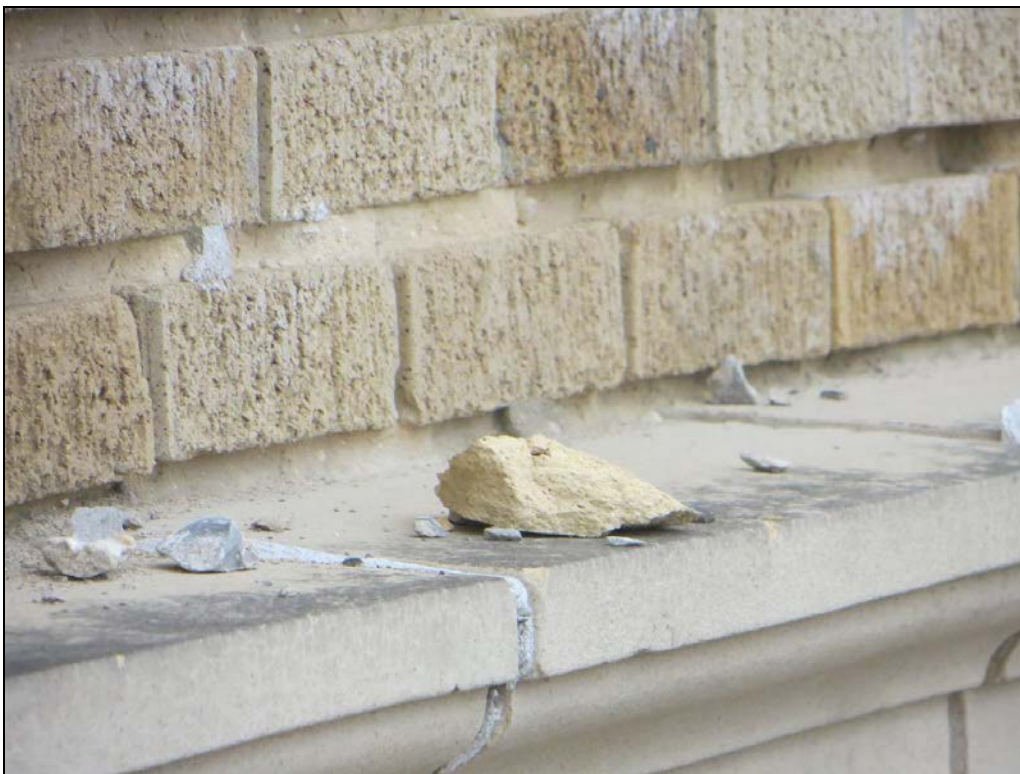
Photograph 24: A piece of terra cotta was found on the smaller terra cotta cornice below.
