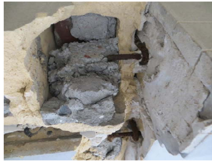
Some heavy surface corrosion was noted on the steel supports, but little loss of cross sectional area was observed.
