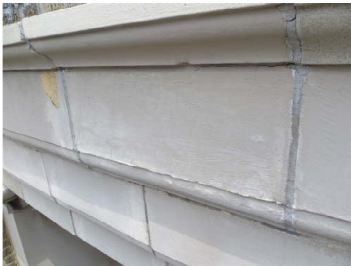
Terra cotta repair mortar appears to be well-bonded to the surrounding substrates.
