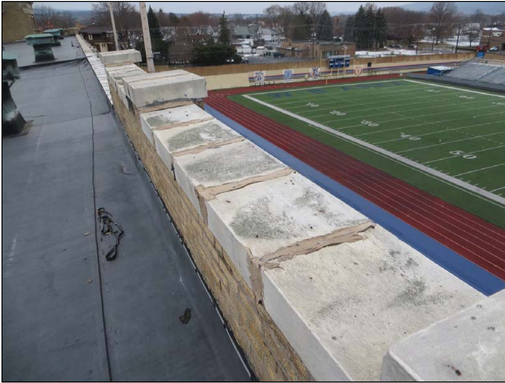
Photograph 29: There was no evidence of flashing under the copings.
