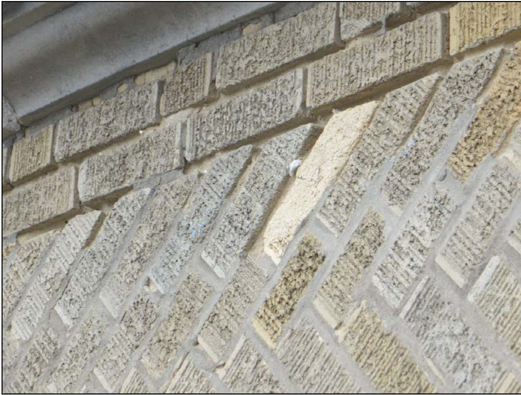
Photograph 13: Open mortar joints at the top of an elevation.
