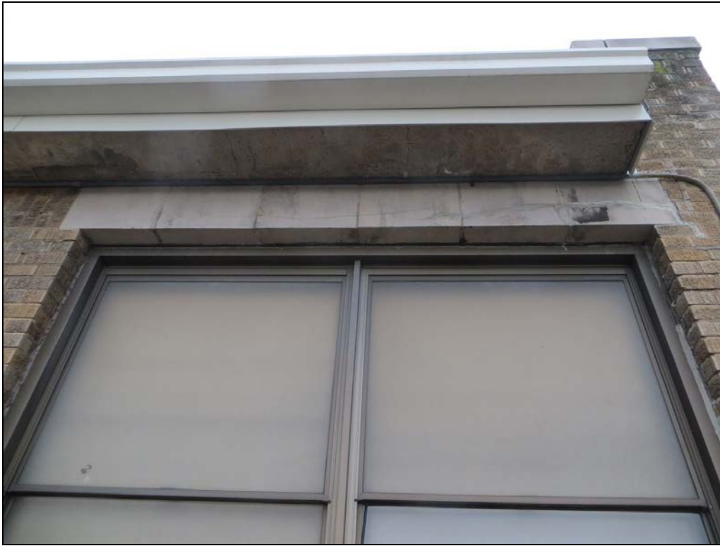
Photograph 31: Cracked terra cotta window header pieces which have been sealed.
