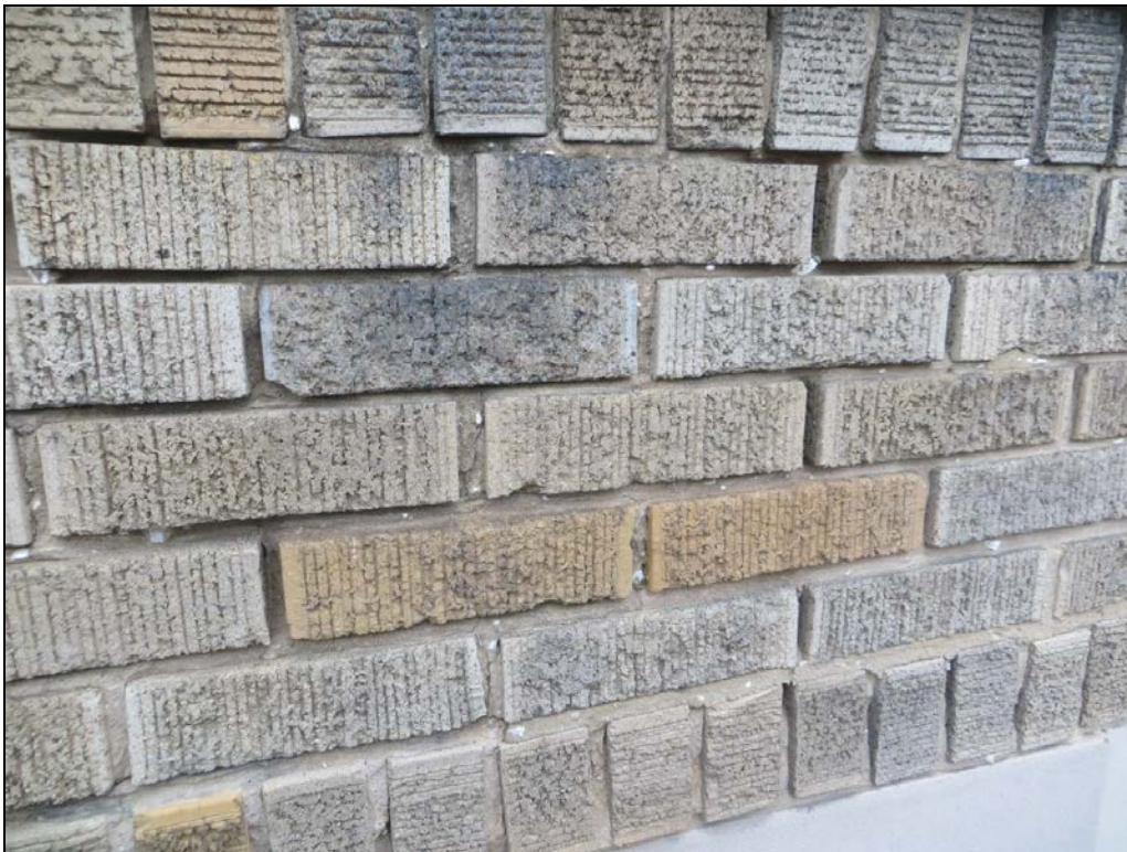
Photograph 14: The original mortar at this location is substantially weathered with numerous failures.
