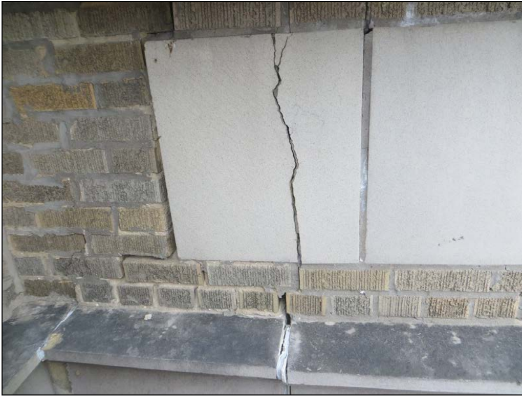
Photograph 27: Crack in a terra cotta panel.
