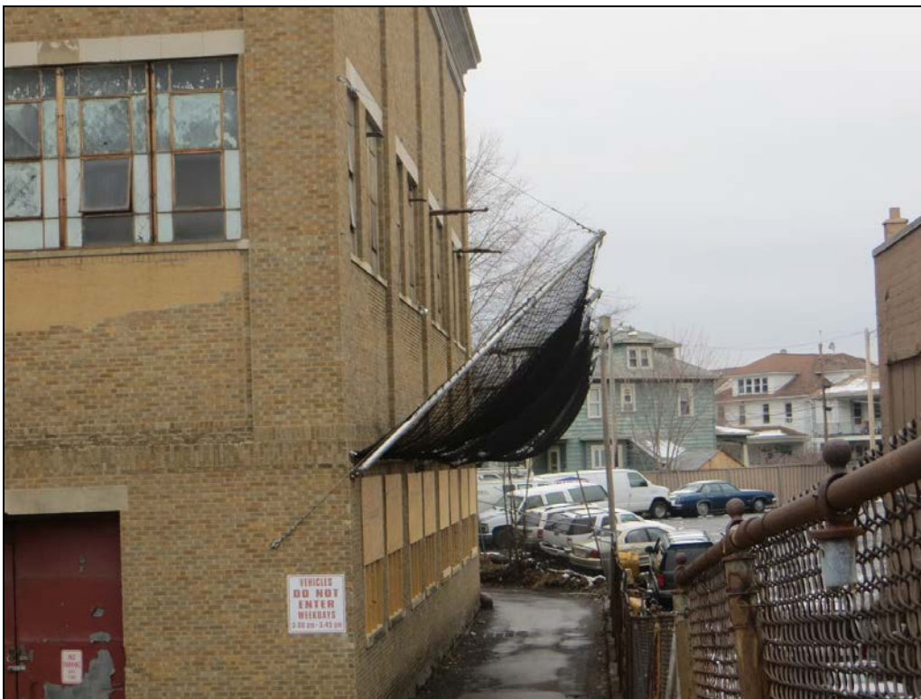
Photograph 54: The deterioration to the mechanical building was so severe extensive netting was required on the north elevation of the building.
