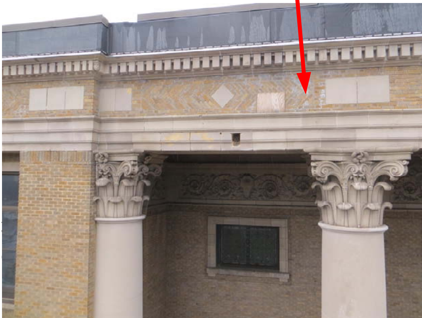
Many of the brick mortar joints had failed, allowing excessive water infiltration.
