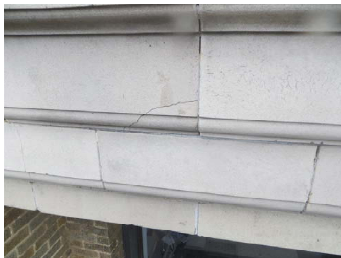
A minor crack in the face of the terra cotta panel.
