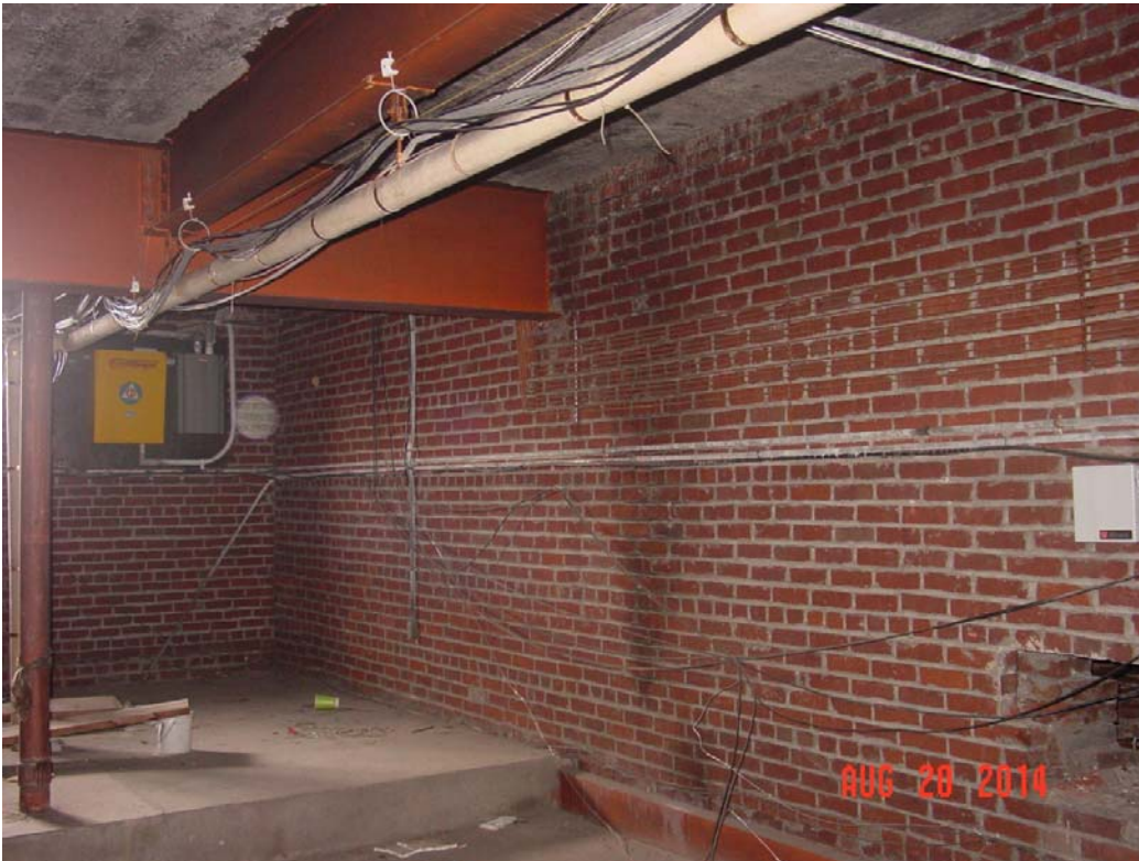
Main Building mechanical room over front entrance. Hole in brick wall allows access to ceiling in Architrave above entrance landing.
