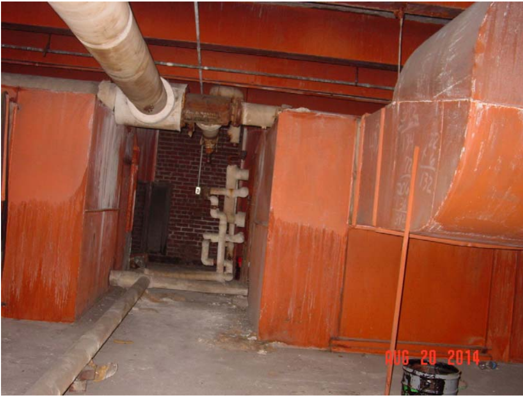
Old mechanical equipment in Mechanical room above Main Building staircase. Floor slopes down 12" to brick wall beyond.
