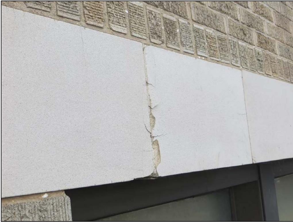
Photograph 39: Spalls on both sides of a mortar joint.
