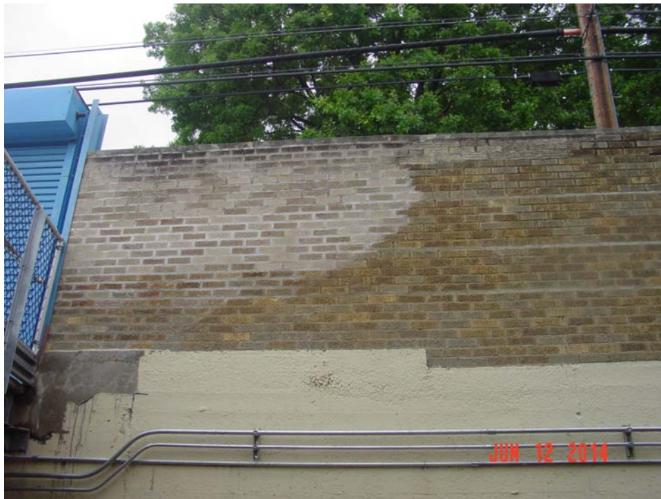
Deteriorated section of brick wall adjacent to Old River Road stadium entrance prior to removal in Summer of 2014
