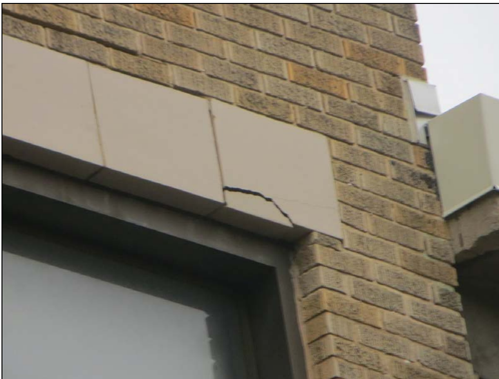
Photograph 36: Spalled terra cotta window header piece.
