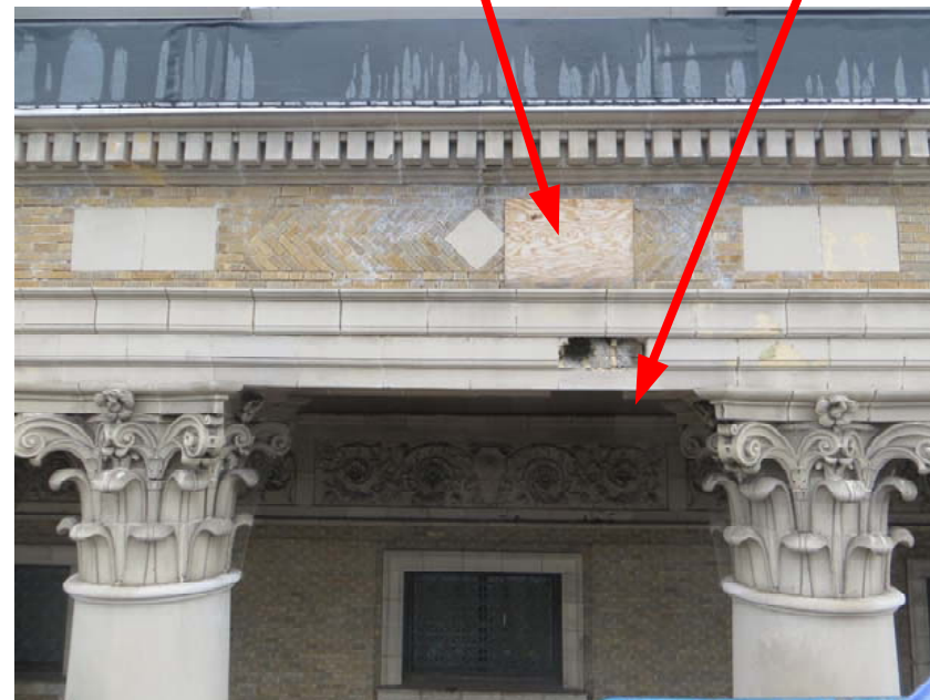
Beam had some surface corrosion but was in good condition.
