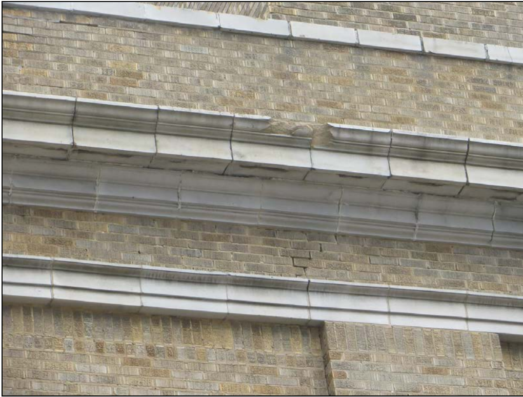
Photograph 53: Large spall in a terra cotta piece at the cornice on the building.
