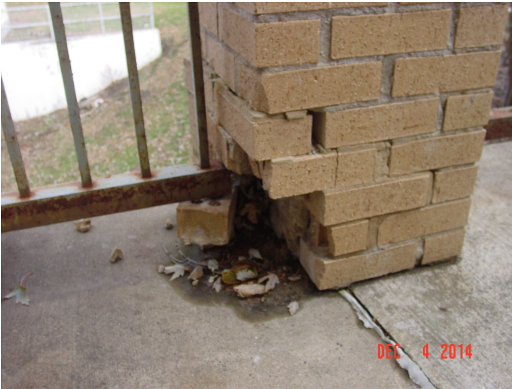
Damaged walkway guardrail. Bottom connection is broken and moves easily. Many other rails are corroded and additional connections may fail in the near future.
