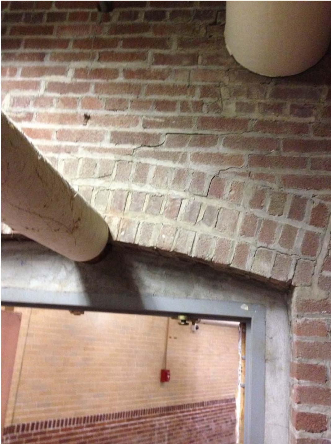
Cracking in basement archway near large pipe penetrations.
