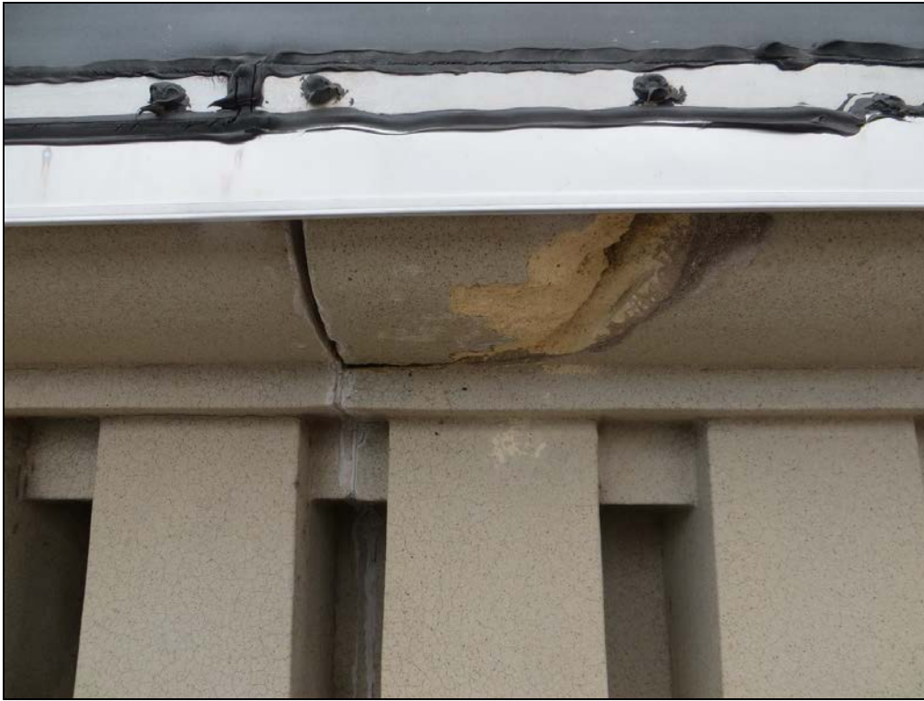
Photograph 23: This spall is loose and being held in place by the metal drip edge.
