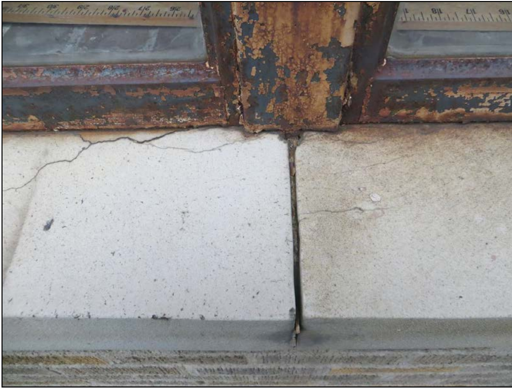
Photograph 43: A cracked window sill caused by a corroded window frame.
