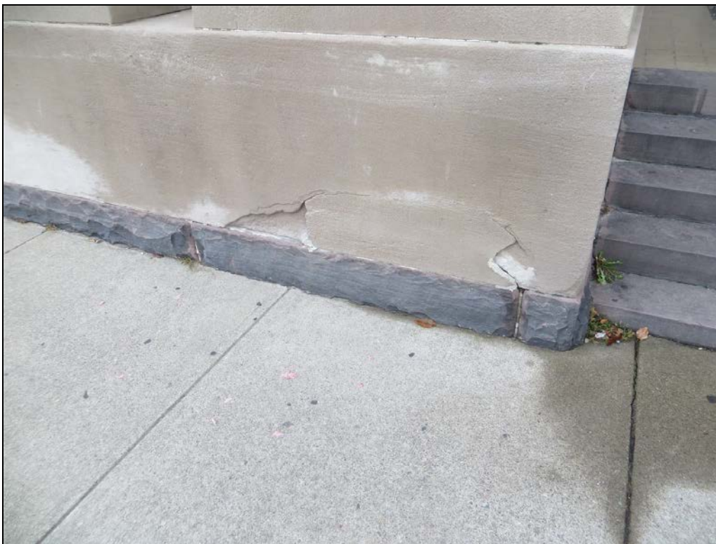
Photograph 46: Spalled limestone piece caused by the use of deicing salts.
