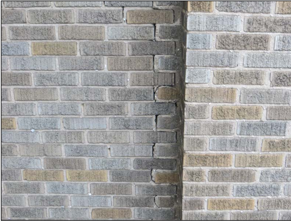
Photograph 17: Cracked mortar at a transition in the brick wall which appears to have been caused by thermal movement in the brick.
