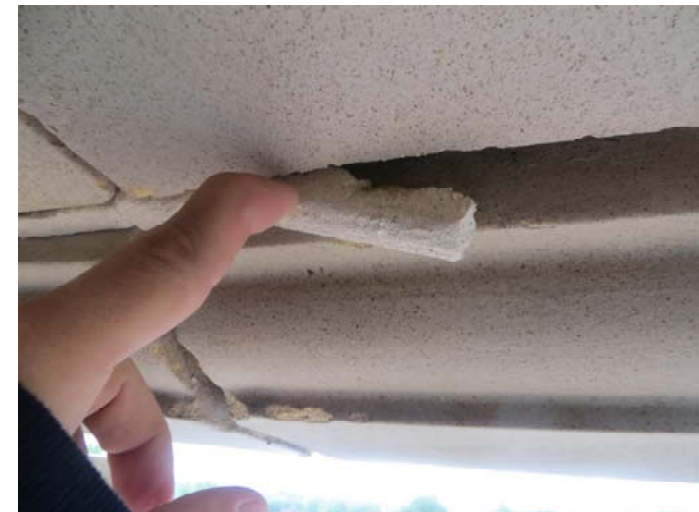
A piece of mortar that was removed by hand with little force used.
