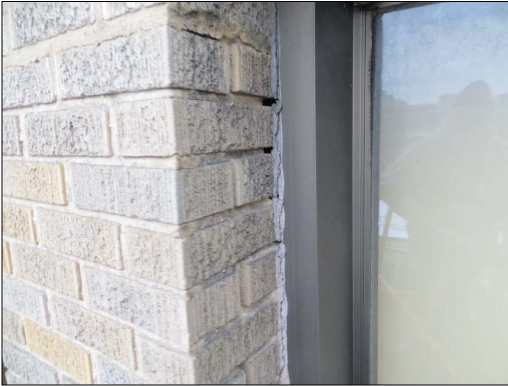
Photograph 49: All of the window sealant appears to have reached the end of its useful life.
