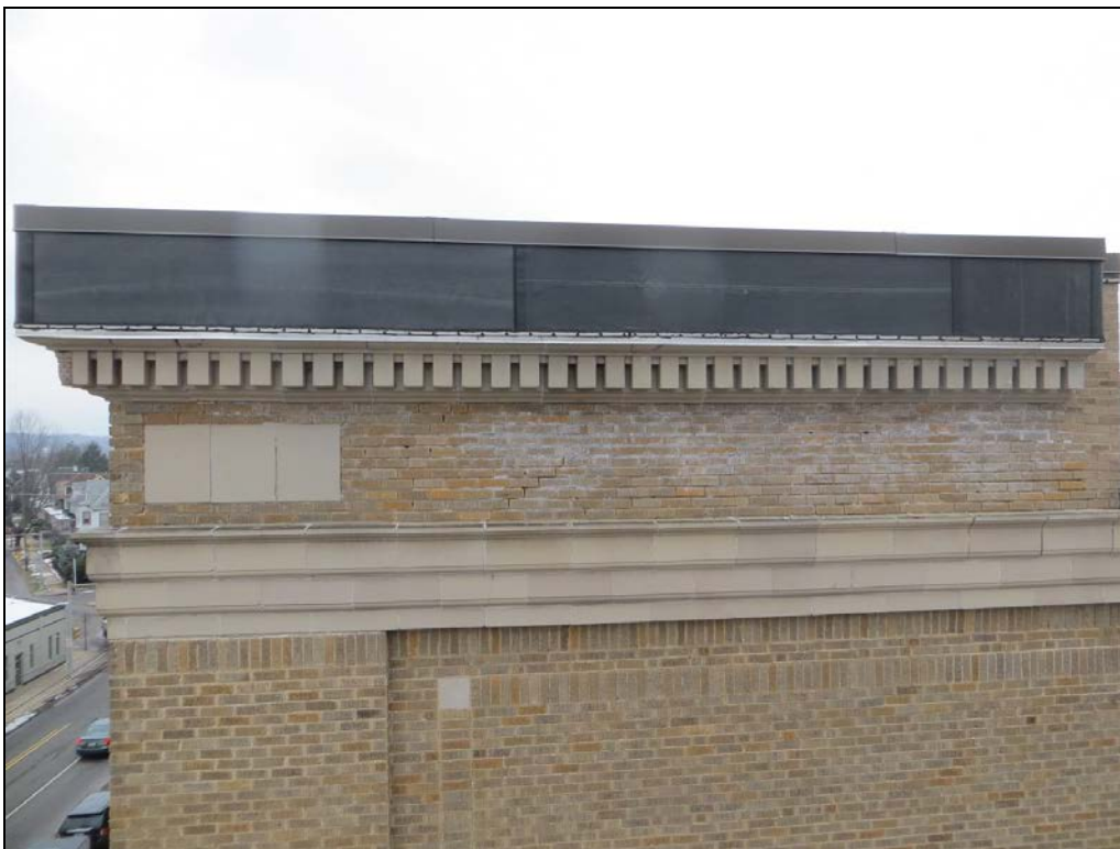
Photograph 8: View of a section of the removed parapet and cornice and the new roofing detail.
