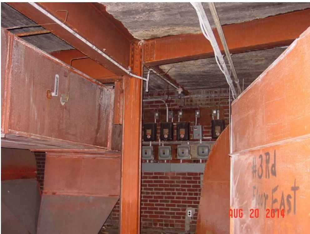
Main Building attic above entrance and central staircase. Note steel beams and column exhibit little to no corrosion.
