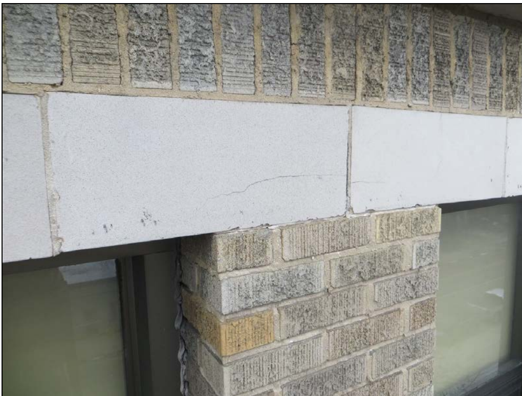
Photograph 32: Cracked window header piece where it is supported by brick.
