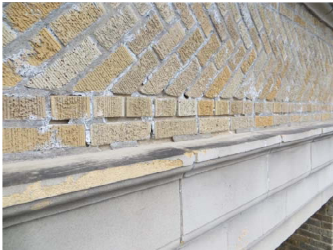
There were numerous failed brick mortar joints.
