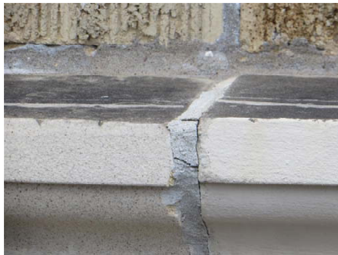
Failed mortar joint adjacent to patched terra cotta piece.
