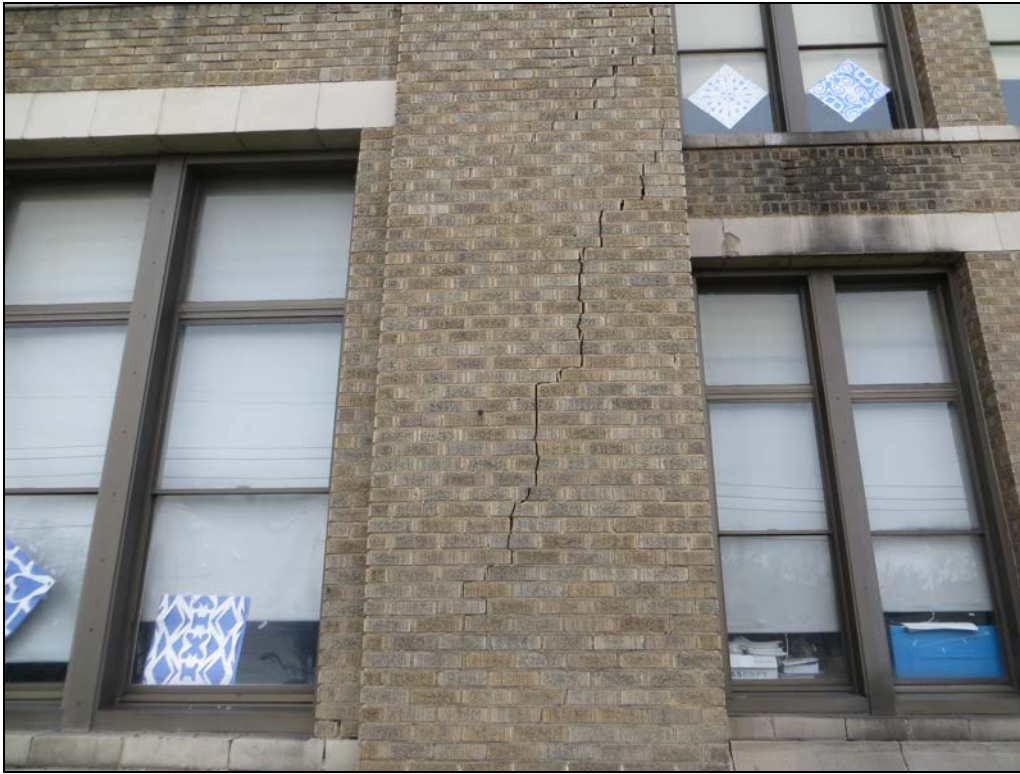
Photograph 19: Significant cracking at a brick pier may have been caused by corrosion of the embedded structural steel.
