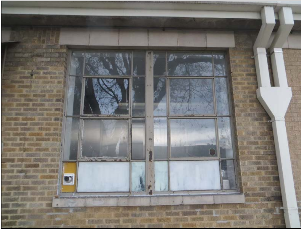
Photograph 55: The original windows on the building are steel framed. These windows are still present at many of the rear elevations.
