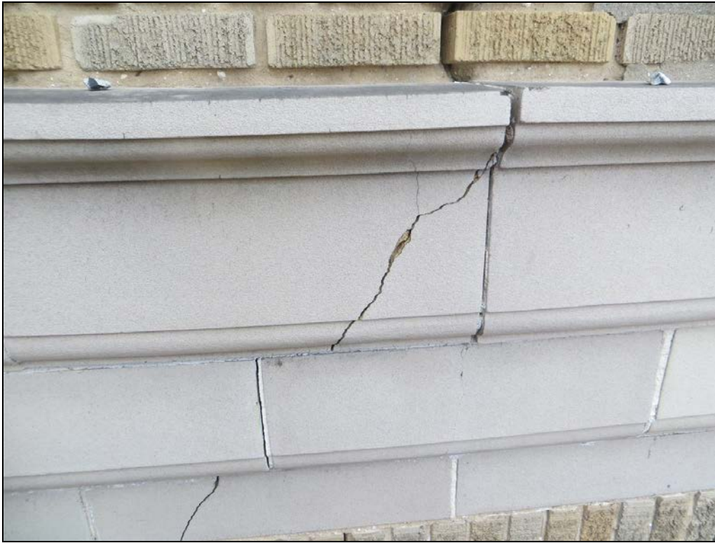
Photograph 25: Crack through the band of terra cotta near the top of the building.
