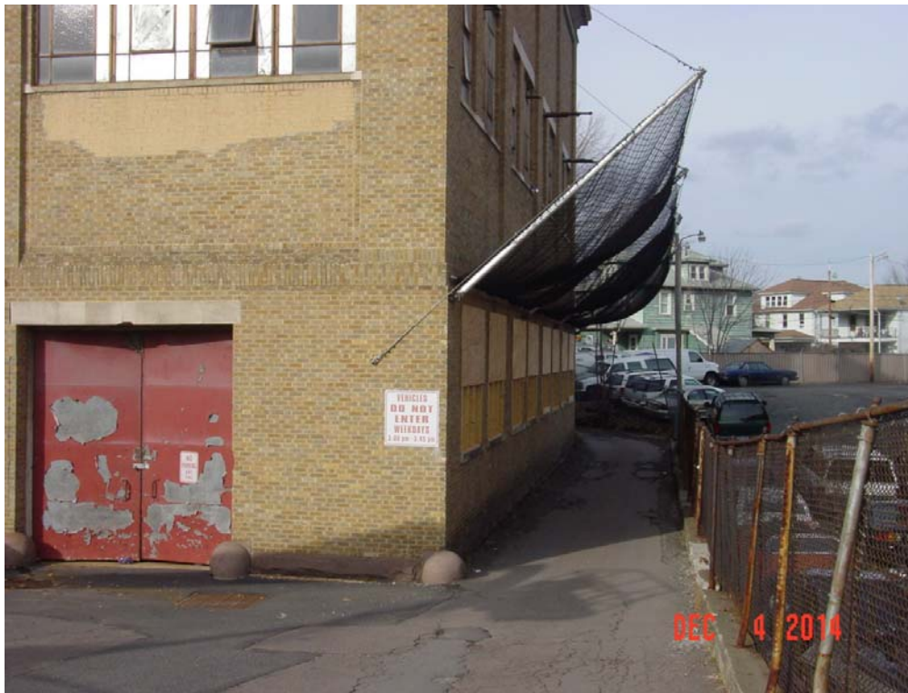
Heating Plant protective netting over Courtyard and Stadium access driveway.
