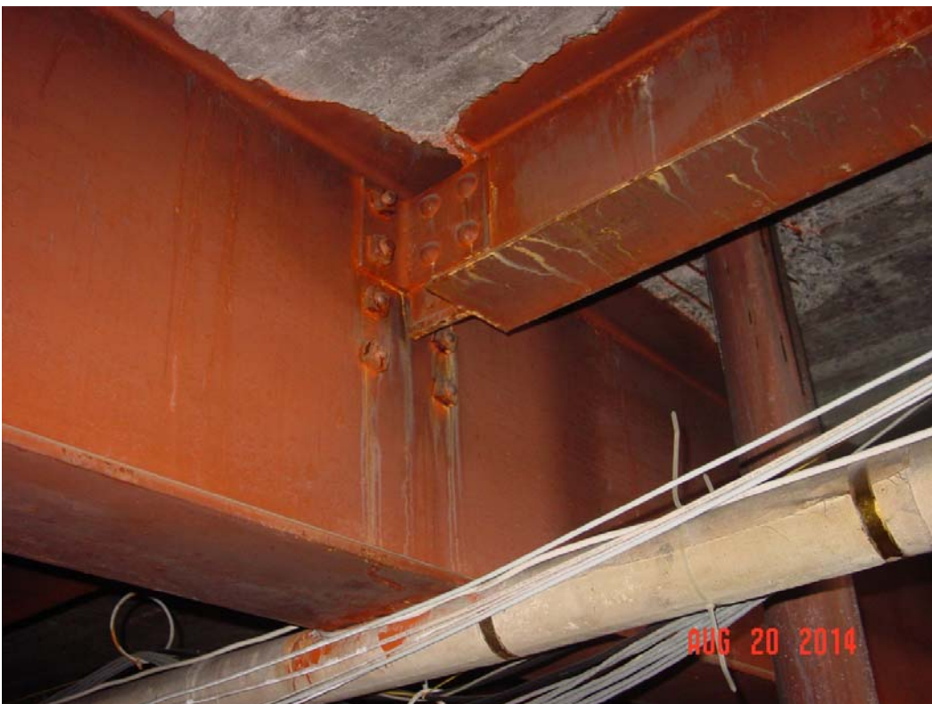
Steel roof beam to girder connection in mechanical room above Main Building staircase
