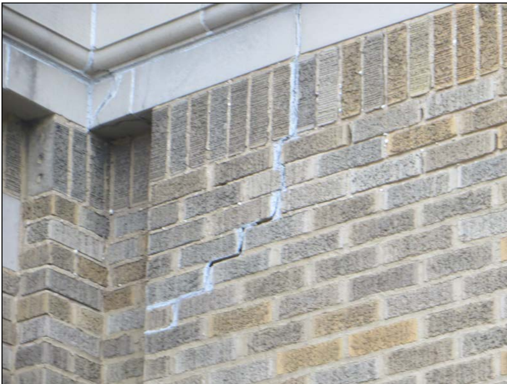
Photograph 20: The crack in the brick continues into the terra cotta.
