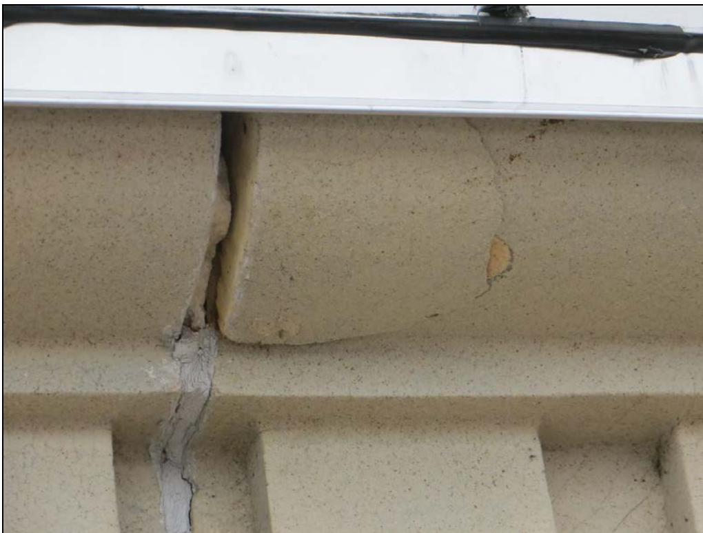
Photograph 22: This insipient spall could come loose at any time.
