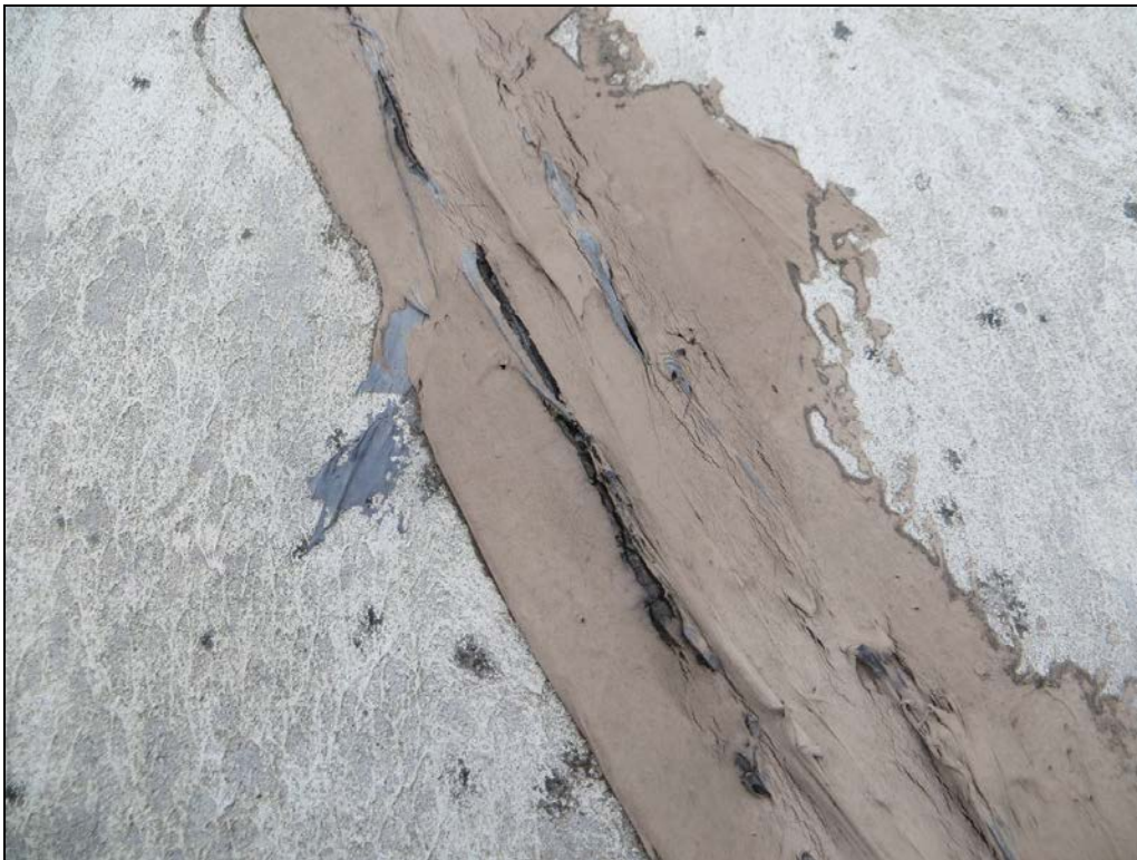
Photograph 30: The joints between the coping pieces had been sealed multiple times, yet we still found multiple failures in the sealant.
