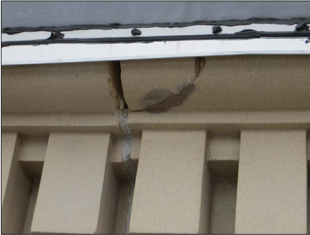
Photograph 21: Spalled terra cotta piece at the top of the elevation. The piece has been poorly repaired and it appears the metal drip edge is the only thing preventing the spall from falling to the ground.
