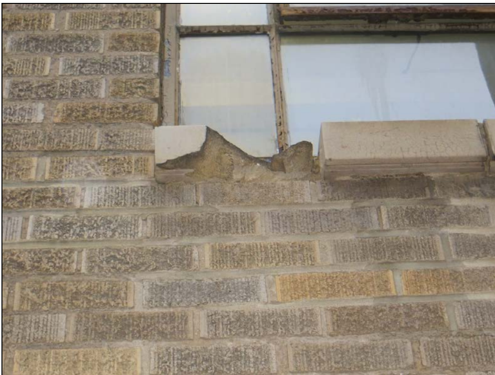
Photograph 44: A terra cotta window sill with significant damage.
