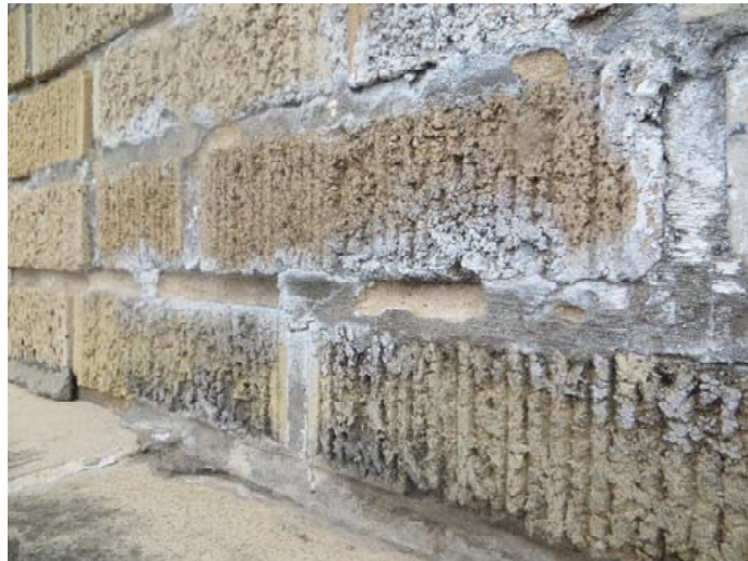
Many of the brick mortar joints had failed, allowing excessive water infiltration.
