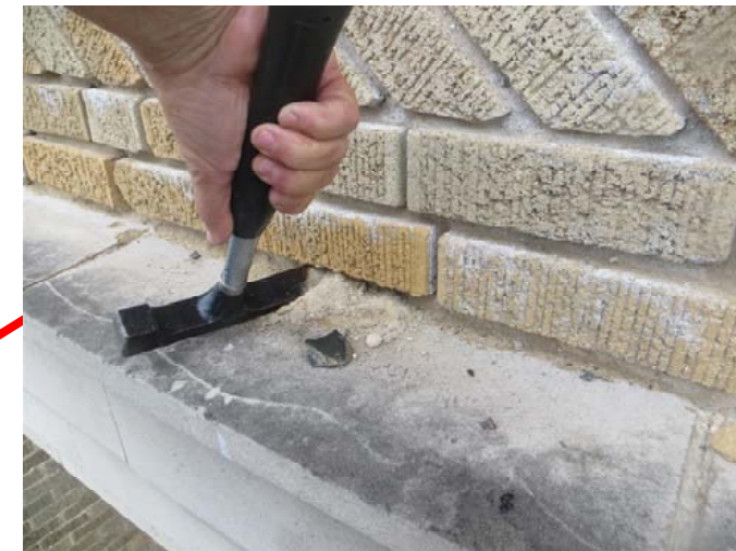
The mortar in the brick above the terra cotta was in poor condition. Previous attempts to repoint the mortar were unsuccessful and have already failed.
