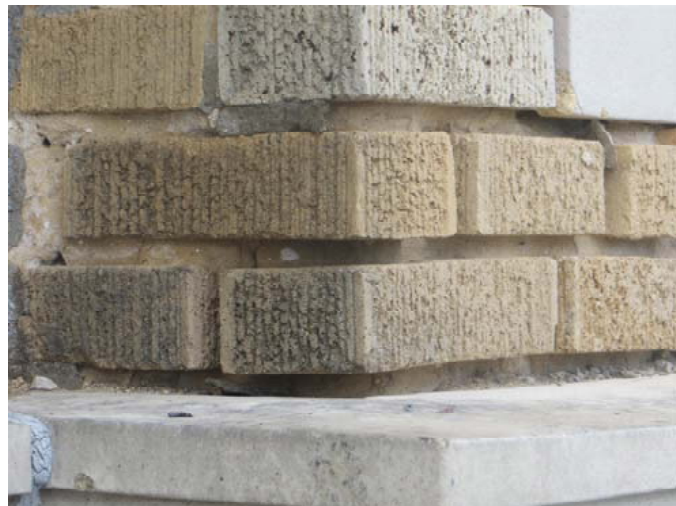
Continued failure of the mortar will eventually compromise the stability of the brick.
