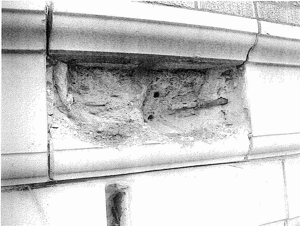
Main Entry - Lower Test Cut
