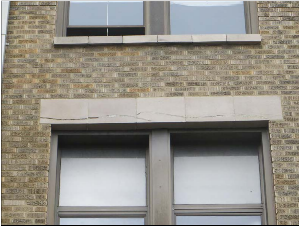
Photograph 35: Crack across all five window header pieces.
