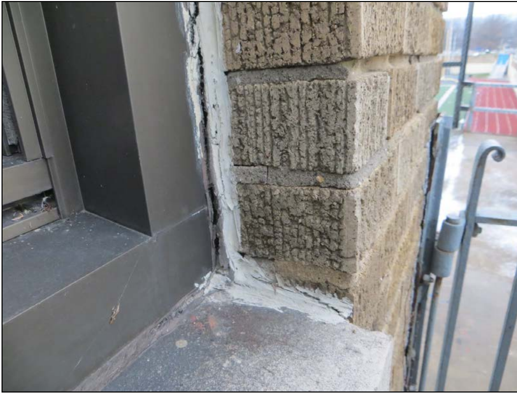
Photograph 47: Failed sealant at the perimeter of a window. There were multiple generations of sealant present.
