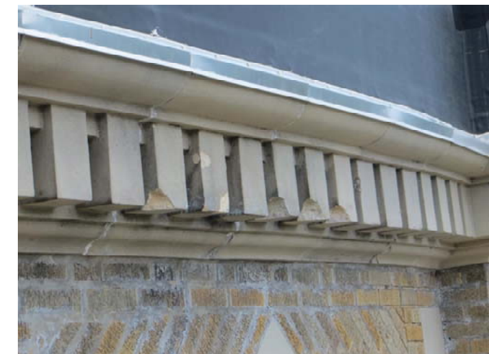
Some small spalls were noted on the dentil above the architrave.
