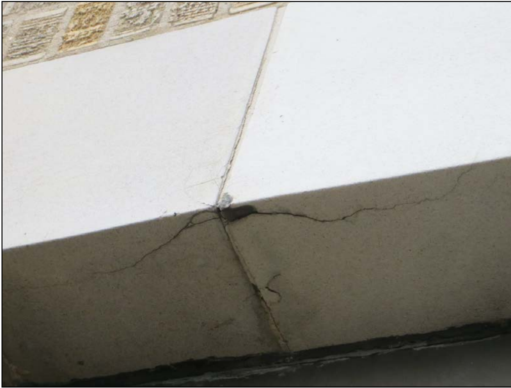
Photograph 33: Crack on the underside of two terra cotta window header pieces.
