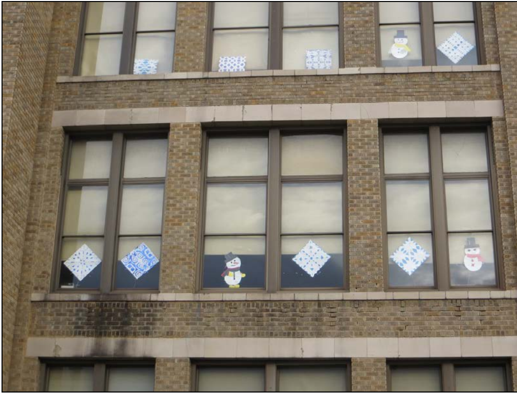
Photograph 7: Typical punched window opening with terra cotta header and sill pieces.
