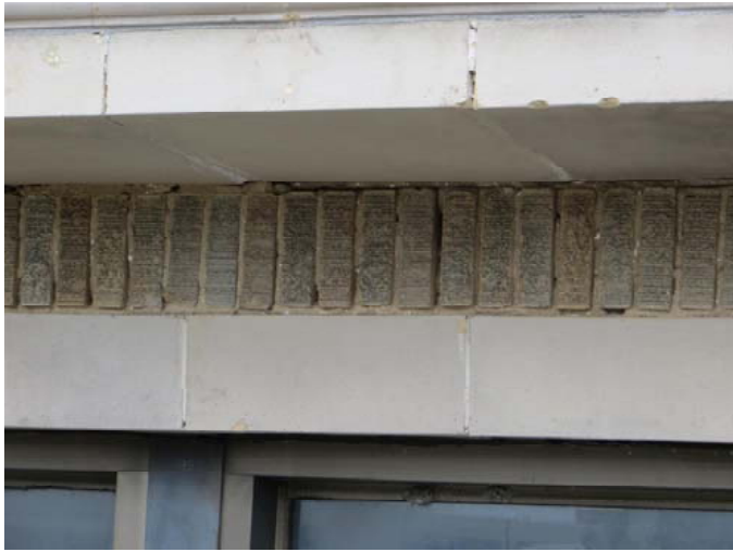
Typical detailing under the terra cotta soffit.
