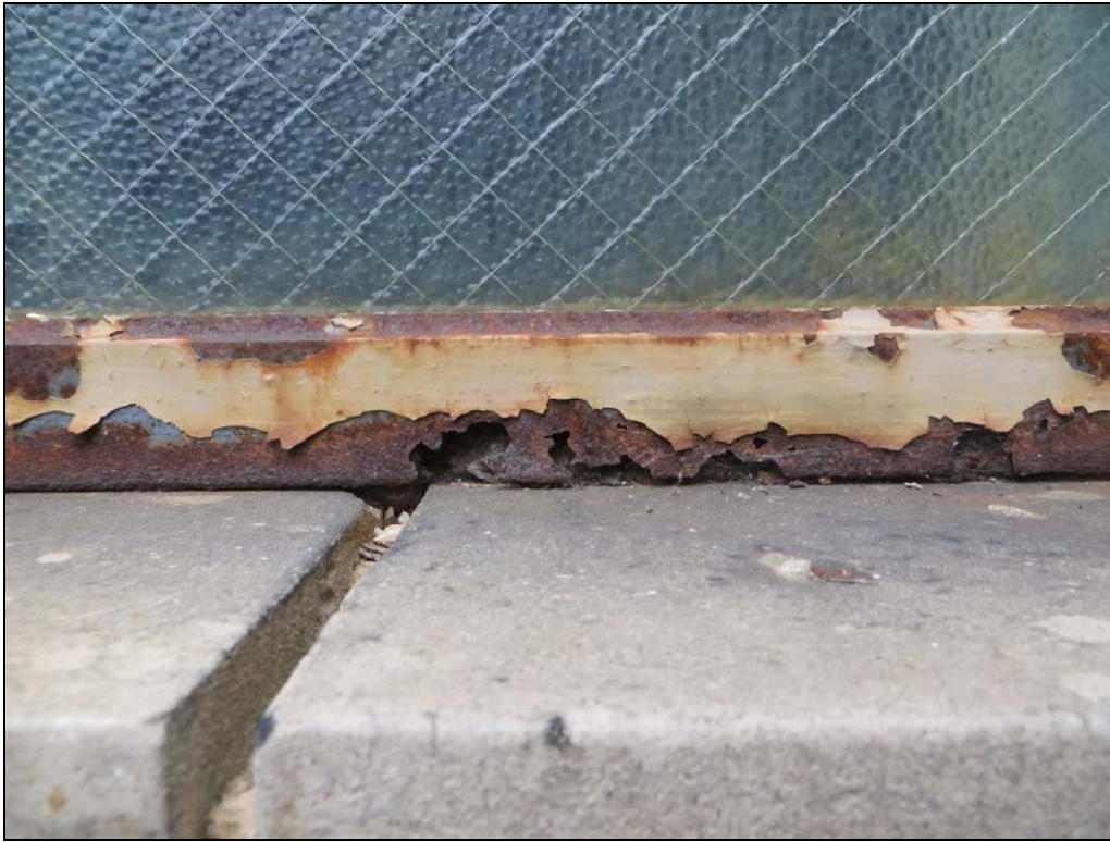
Photograph 57: Several of the remaining steel framed windows are heavily corroded.
