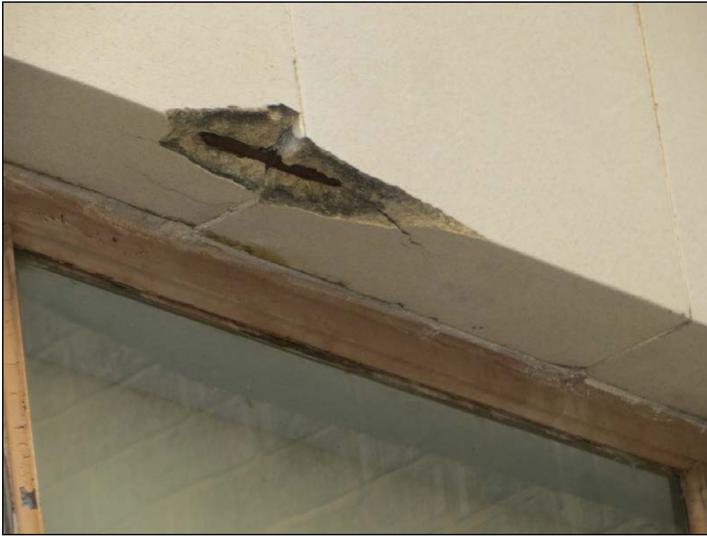
Photograph 37: Spall at corroded pin between pieces.
