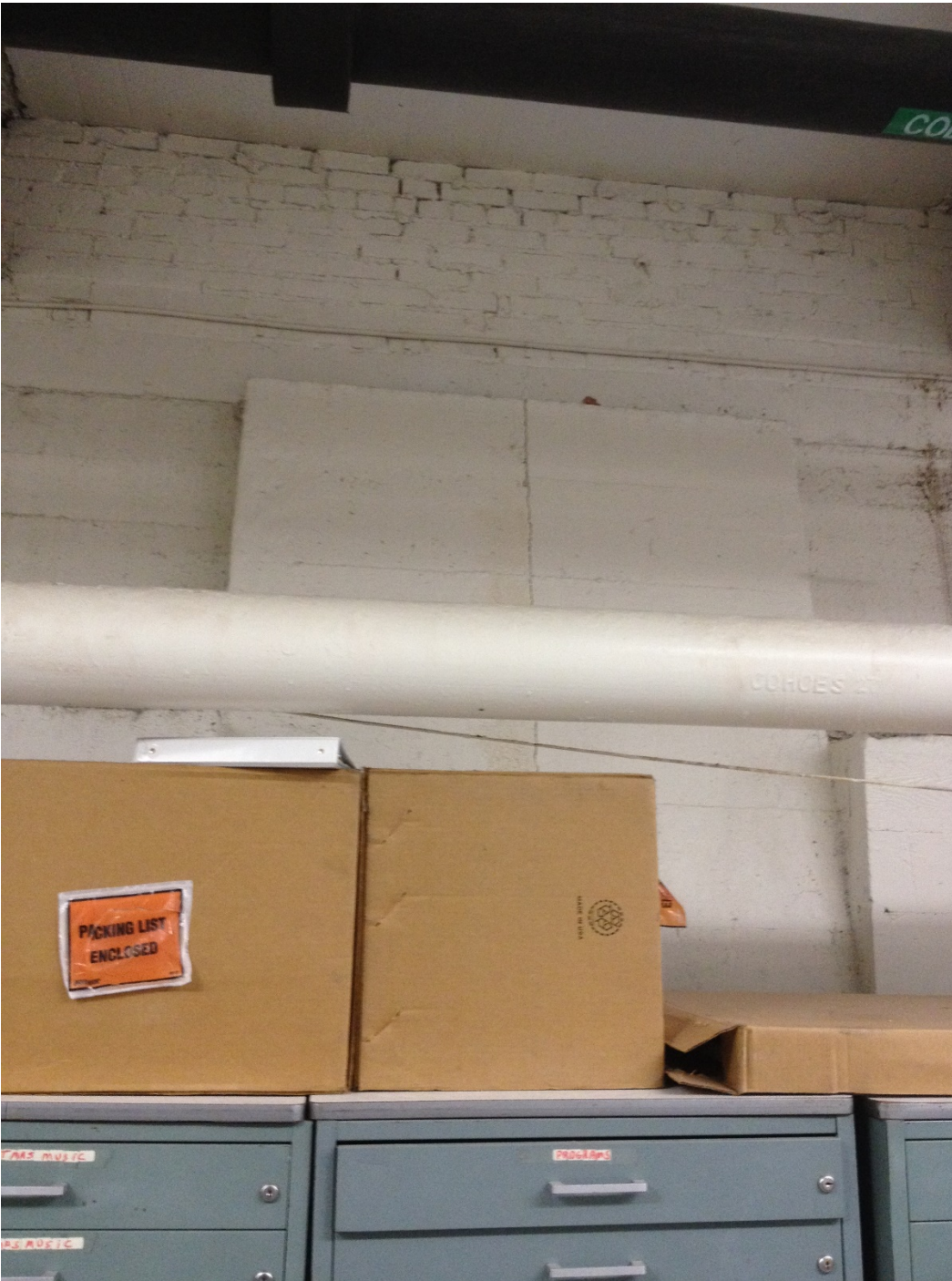
Mass concrete retaining wall below base of exterior brick wall.
