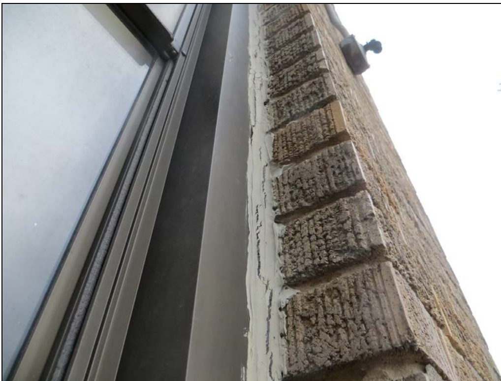
Photograph 48: This sealant joint had both adhesive and cohesive failures.
