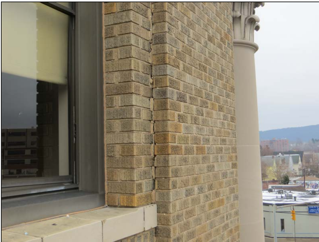
Photograph 18: Cracked brick where the brick sets back at a window. This also appears to have been caused by thermal movement of the brick.
