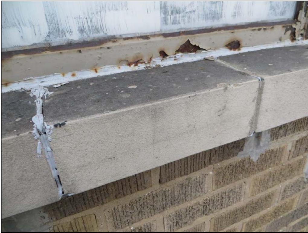
Photograph 41: The joints between the window sill pieces were in poor condition.
