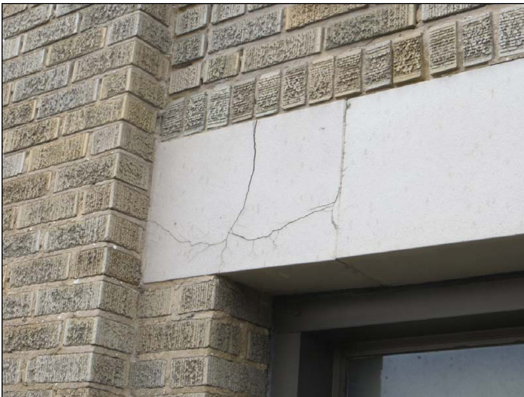
Photograph 34: Multiple cracks in one window header piece.
