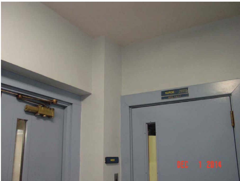
First floor interior corner at entrance to Main Building staircase from corridor running parallel with Carey Avenue. The Floor slopes 12" from front to rear in this area.
