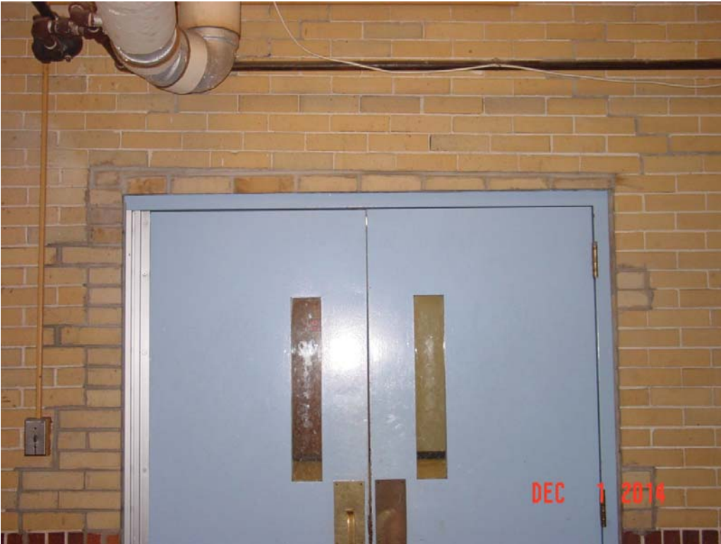
Door leading into basement level of Main Building staircase. Note the slope of the brick above door.
