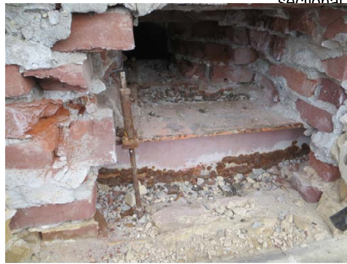
Beam had some surface corrosion but was in good condition.
