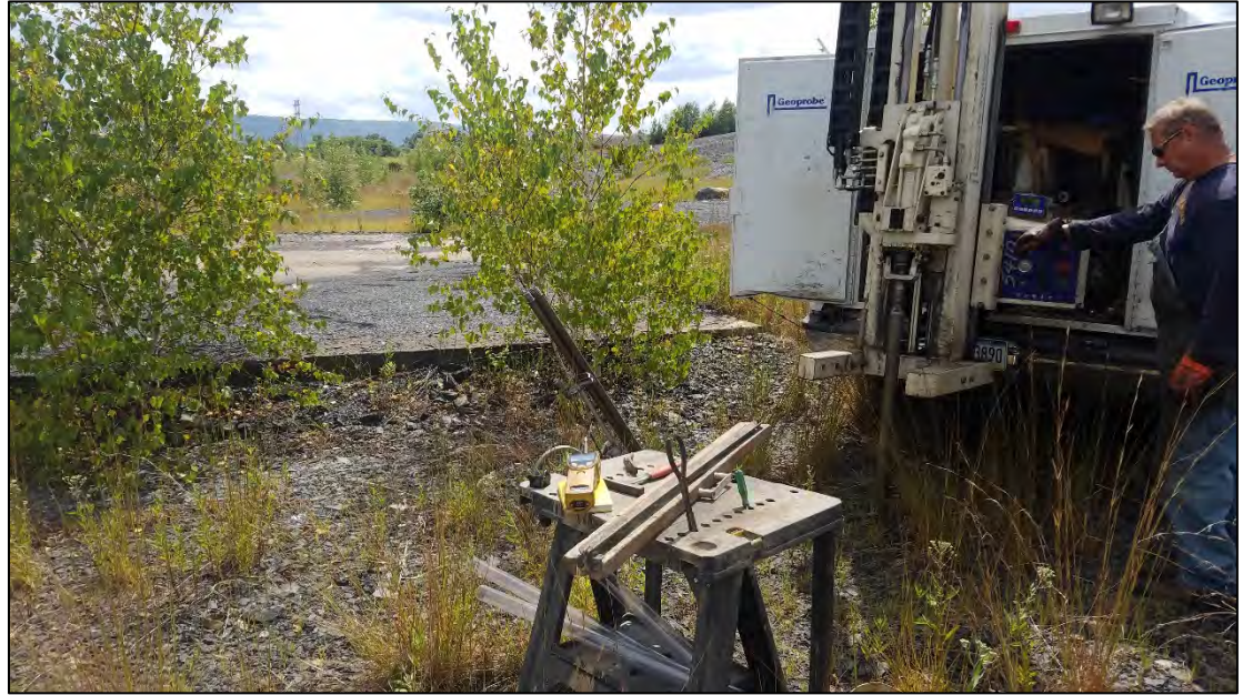
Photo 9. View of SB-035 in progress. SB-034 and SB-035 were completed adjacent to the concrete slab.
