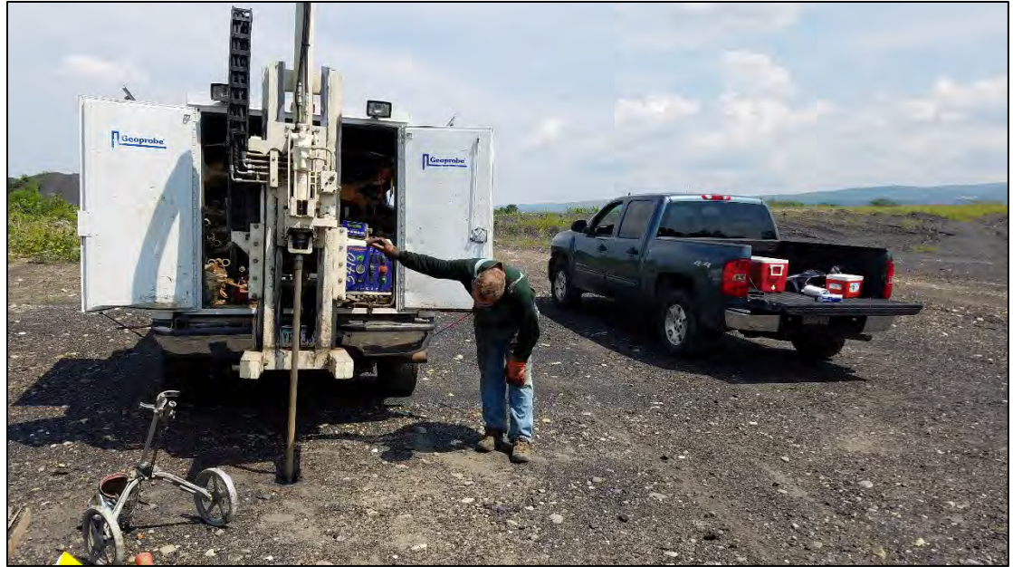
Photo 3. View of Geoprobe installing a soil boring. Typical of all borings. Photo taken August 2017.
